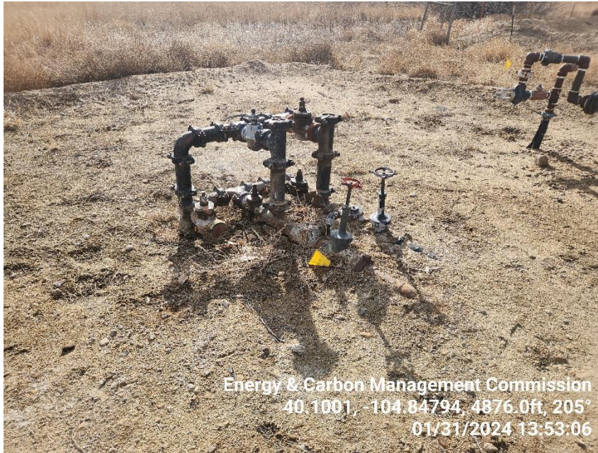
Photo 5 Flow line manifold.
