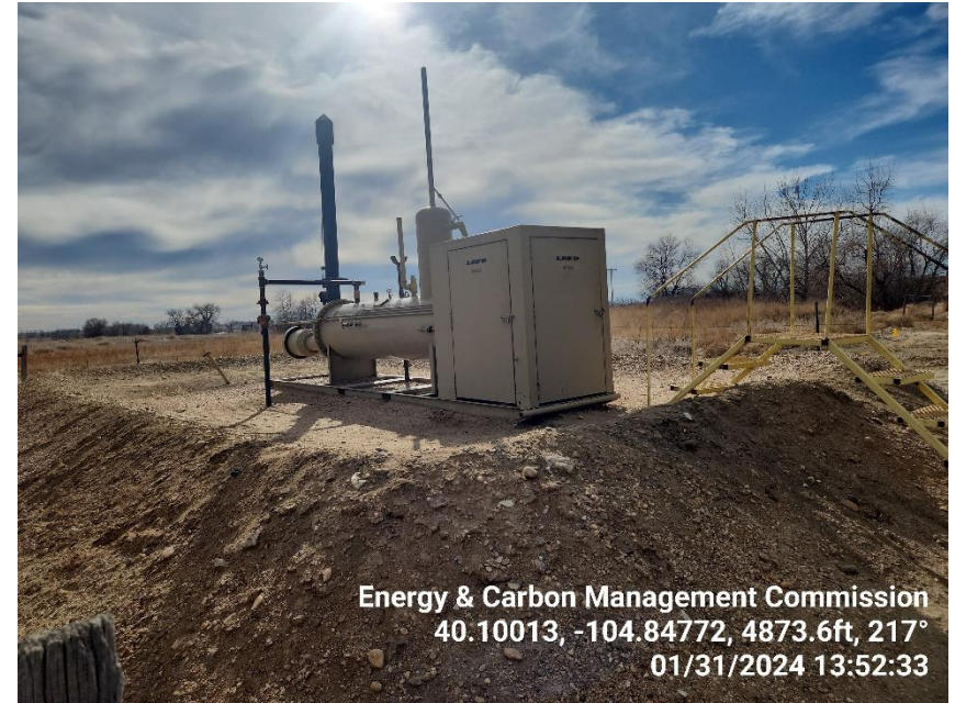
Photo 6 Horizontal Heated Separator.
