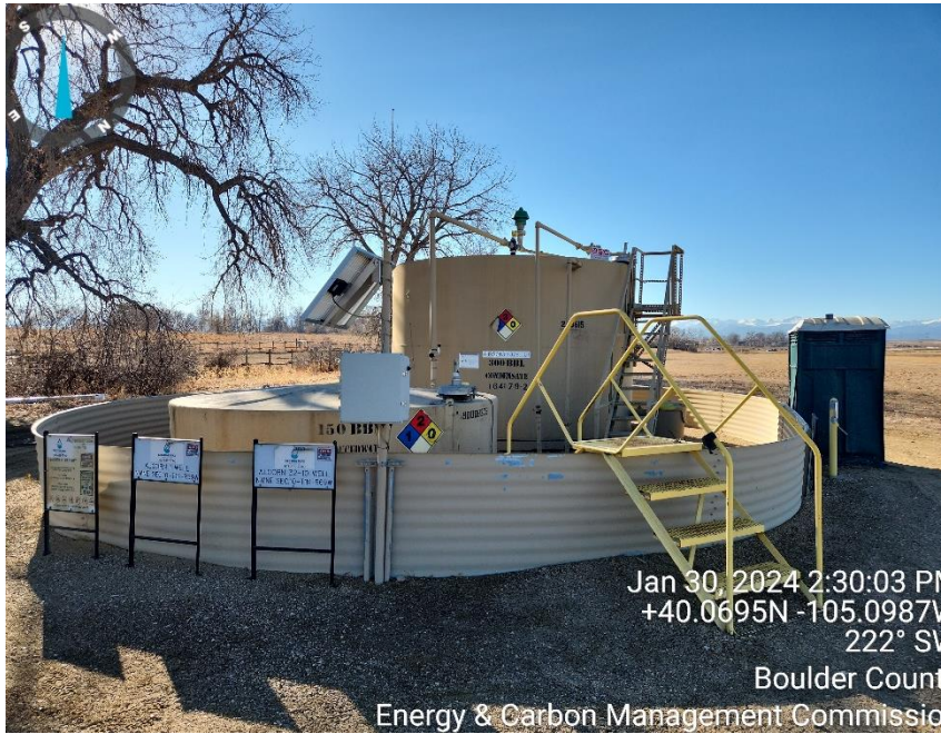
Photo 3 tank battery
