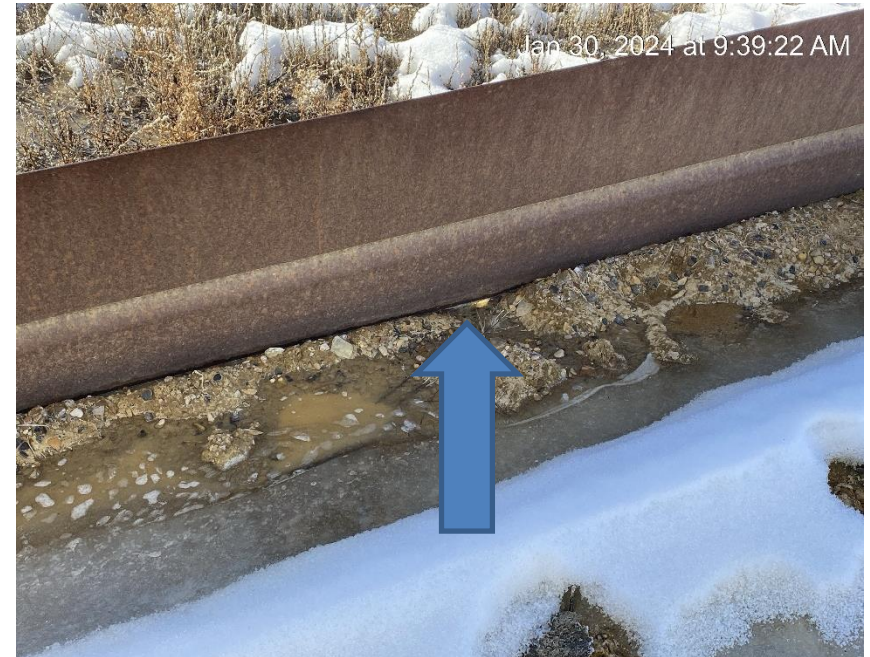
Metal tank berm leak
