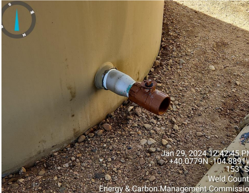
Photo 9 water tank valve need plug
