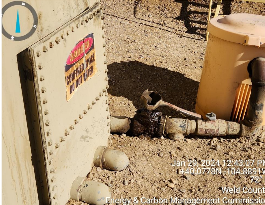
Photo 11 plug valve on SE oil tank
