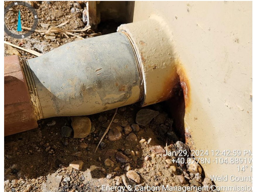
Photo 10 leak on water tank drain valve
