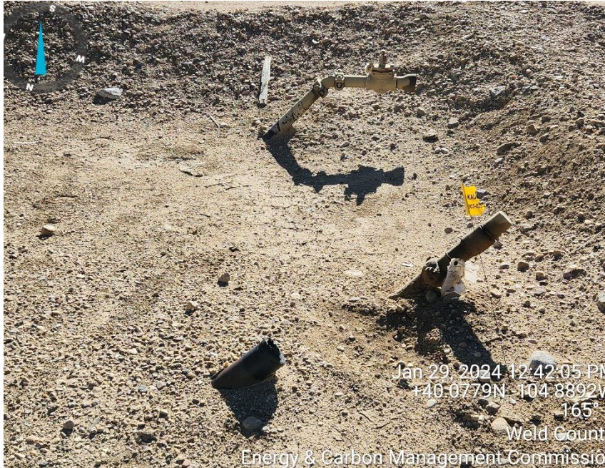
Photo 5 riser in tank berm not ID or tagged
