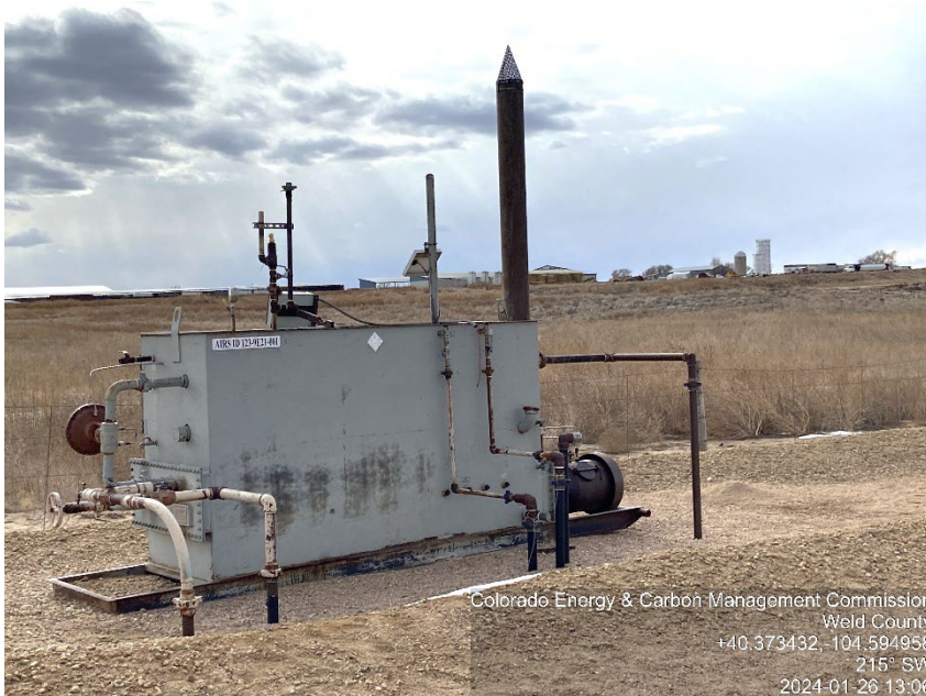
Photo #3 Lion #2 Battery site Active Separator(s)
