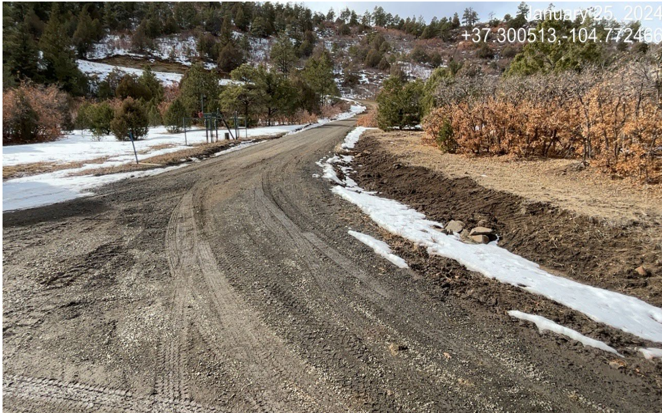
Photo 3. Facing southwest along. There has been repairs performed along the road and disturbed areas were seeded.
