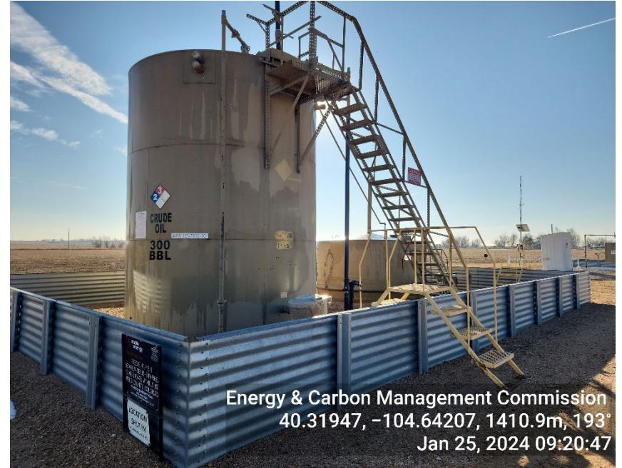
Photo 2: Tank Battery
