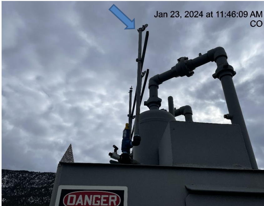
Photo # 3445 Cap installed on PRV vent line by Caerus employee
