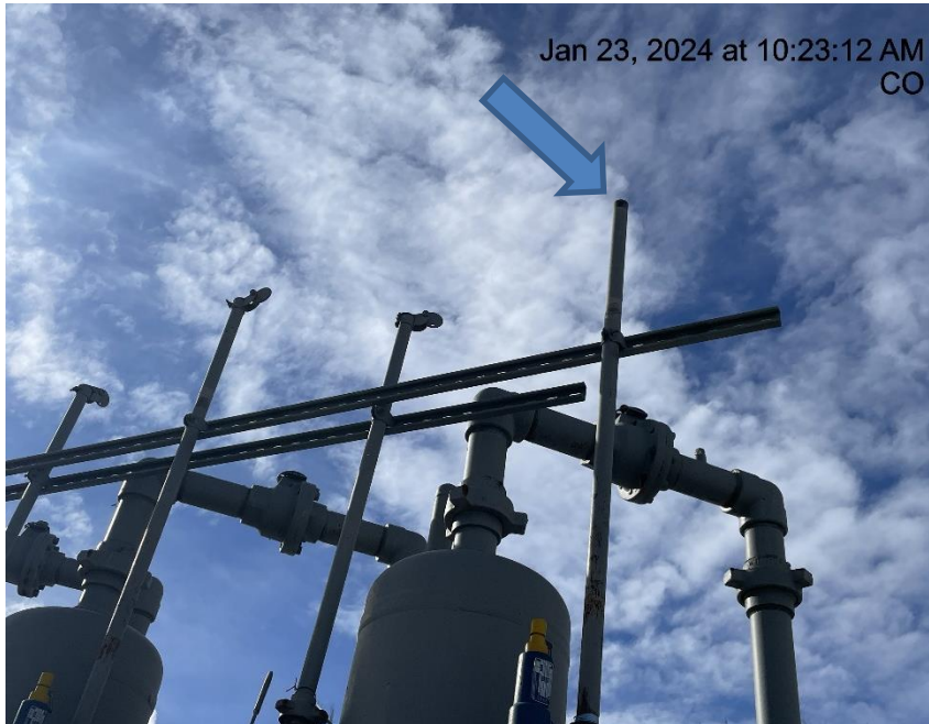
Photo # 3443 PRV vent line lacks cap
