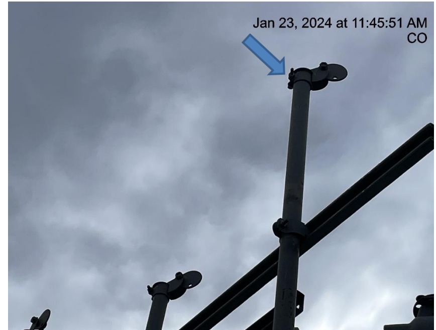
Photo # 3446 Cap installed on PRV vent line by Caerus employee
