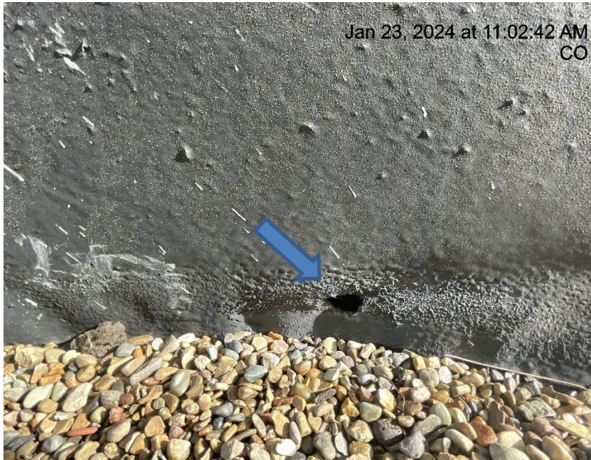
Photo # 3496 Hole in secondary containment liner
