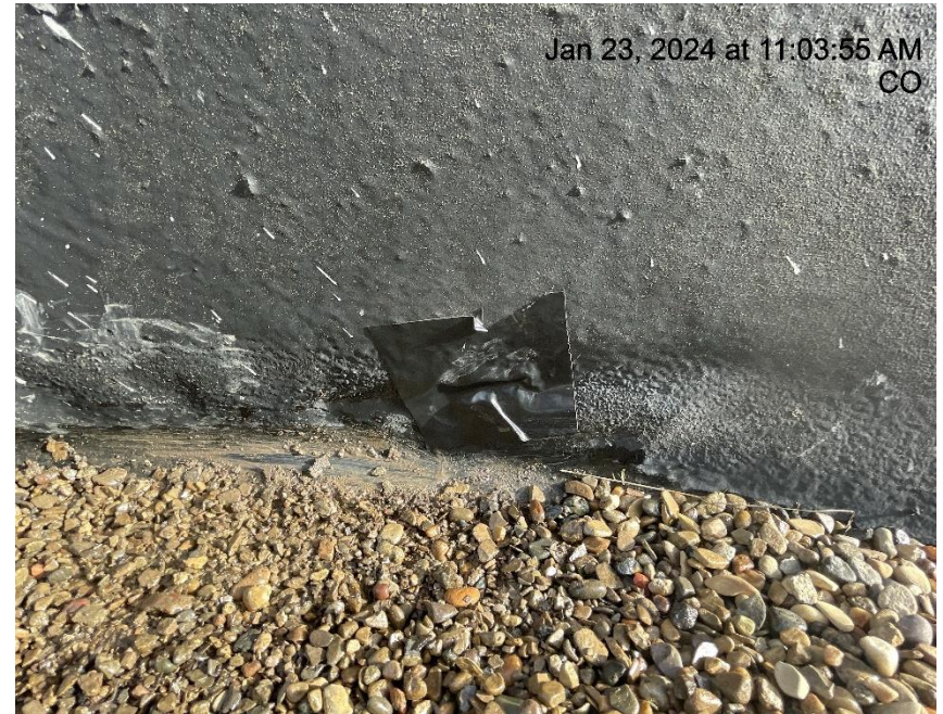
Photo # 3497 Hole patched by Caerus employee during inspection
