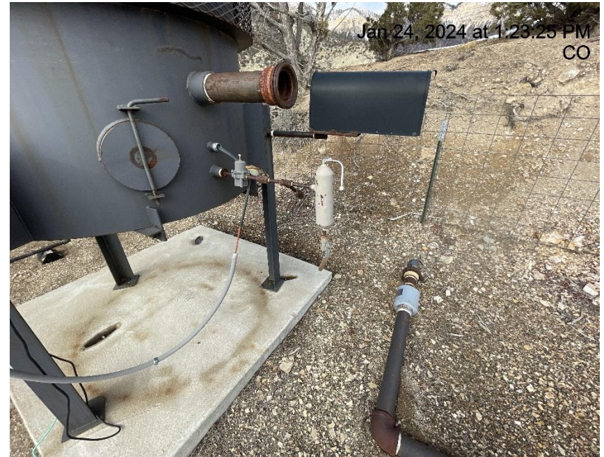
Photo # 3790 Unused equipment/ESD disconnected
