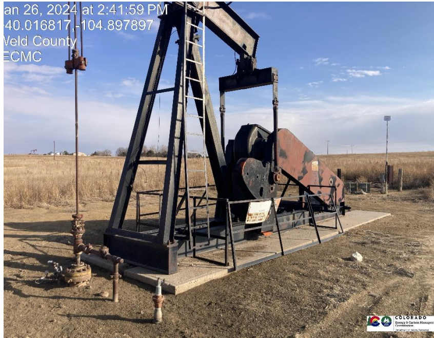
Pic 1 wellhead / pumpjack
