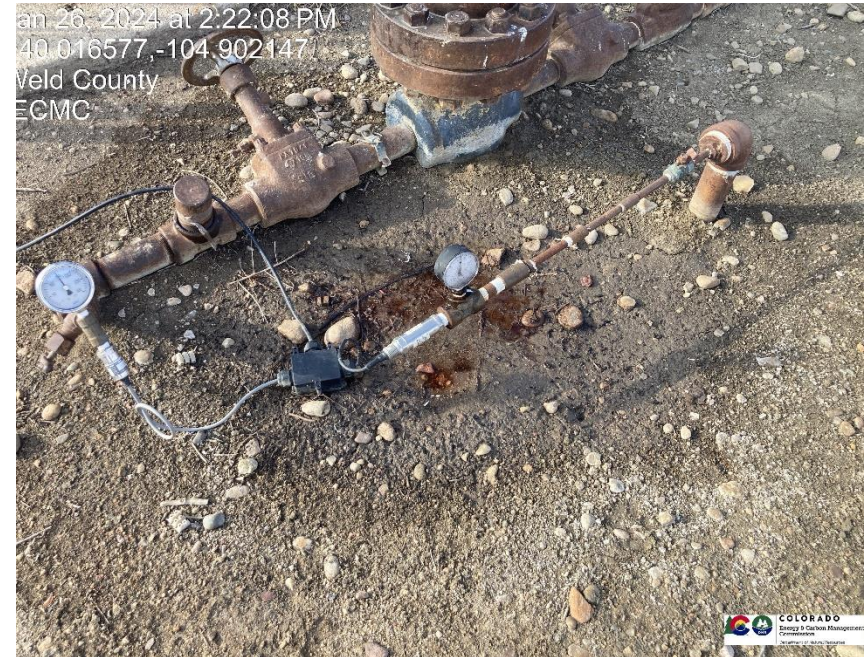
Pic 2 leak on piping for bradenhead, gauge shows 17 PSI on bradenhead.
