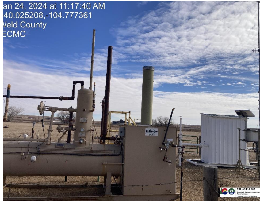
Pic 1 Separator, ECD, GMR
