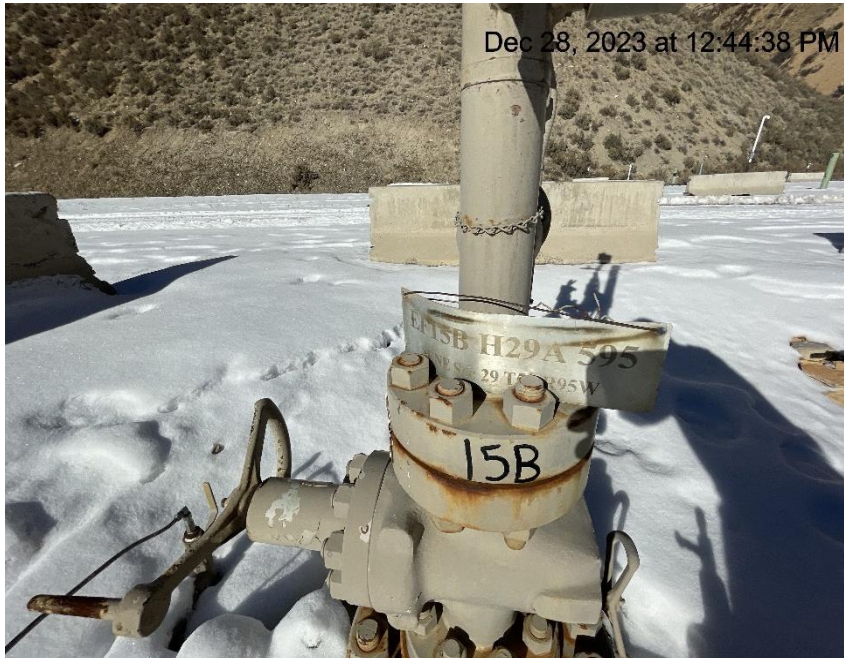
Photo # 1208 From inspection 708902630 conducted on 12/28/2023 All wellhead signs on location lack required information/wellhead signage insufficient/signs are not in compliance with CECMC rules
