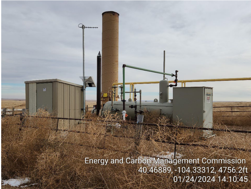
Photo 1 – Separator, ECD and Gas Meter – Weeds
