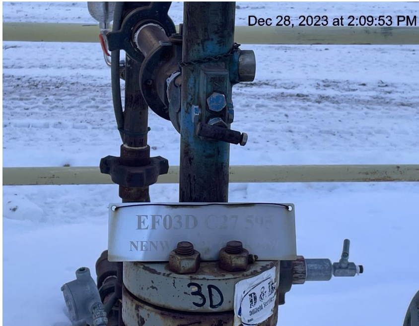
Photo # 1369 From inspection 708902651 conducted on 12/28/2023 Wellhead sign lacks required info/sign in not in compliance with CECMC rules
