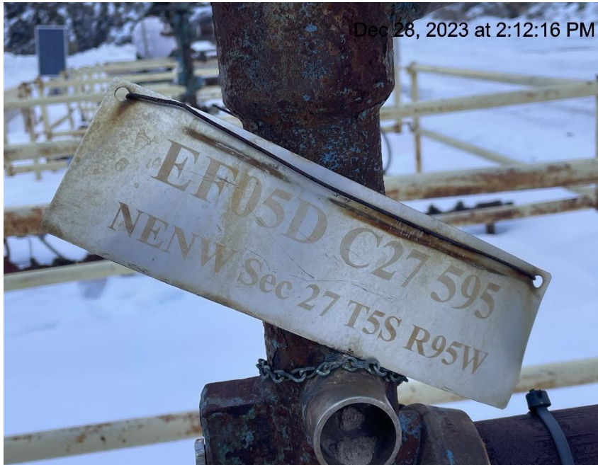
Photo # 1368 From inspection 708902651 conducted on 12/28/2023 Wellhead sign lacks required info/sign in not in compliance with CECMC rules
