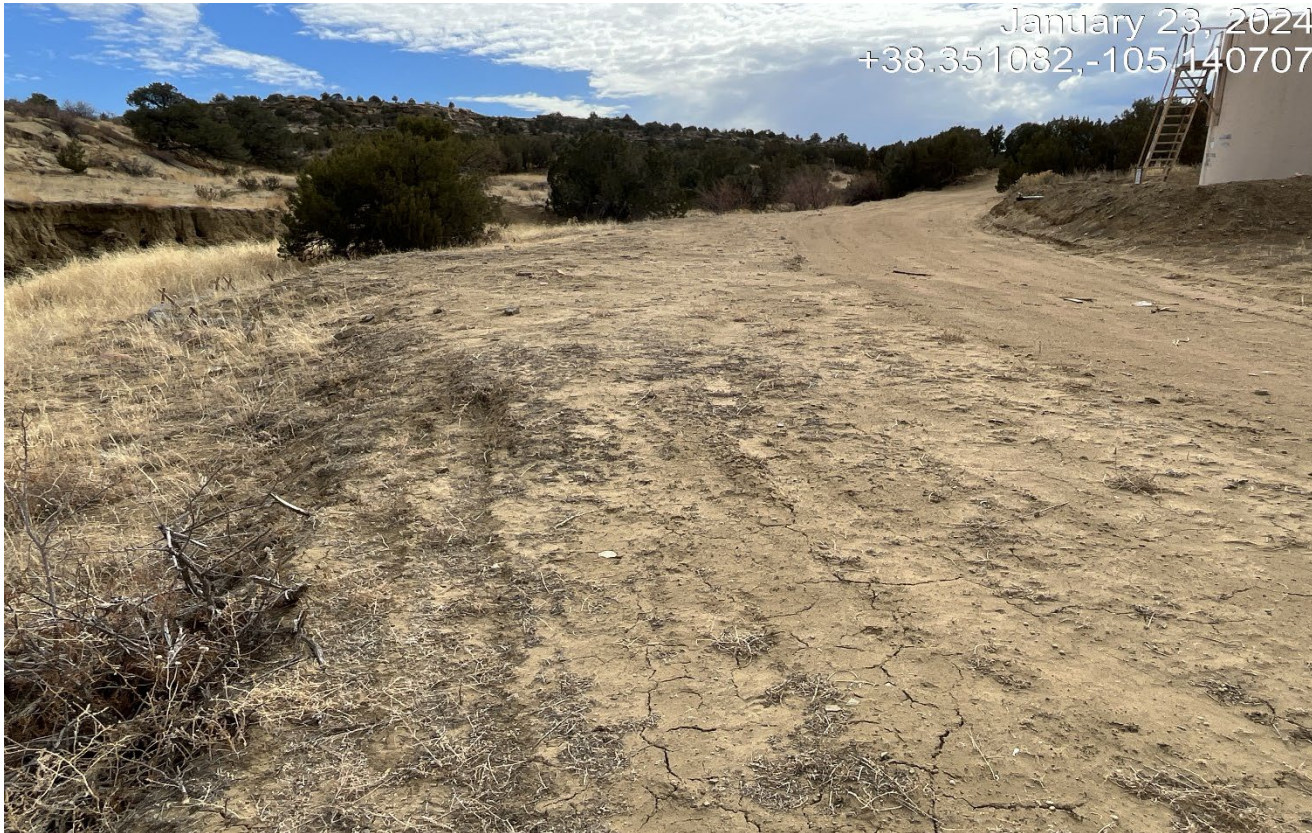
Photo 6. Facing southeast at the tank battery site. The disturbed area along the road side needs to be reclaimed and stabilized. Previous corrective action was not completed.
