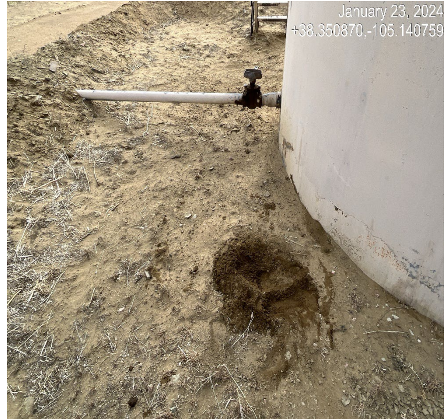
Photo 10. There appears to be oil stained soil at the from side of the tank.
