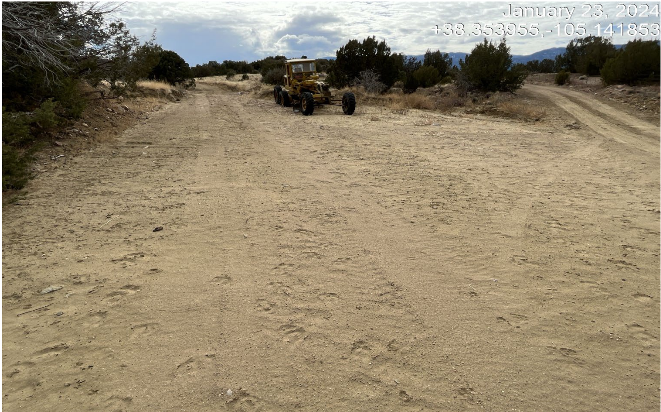
Photo 1. Facing southeast along the access road. This area has been regraded since the previous inspection. The sandy loose soils need to be stabilized.
