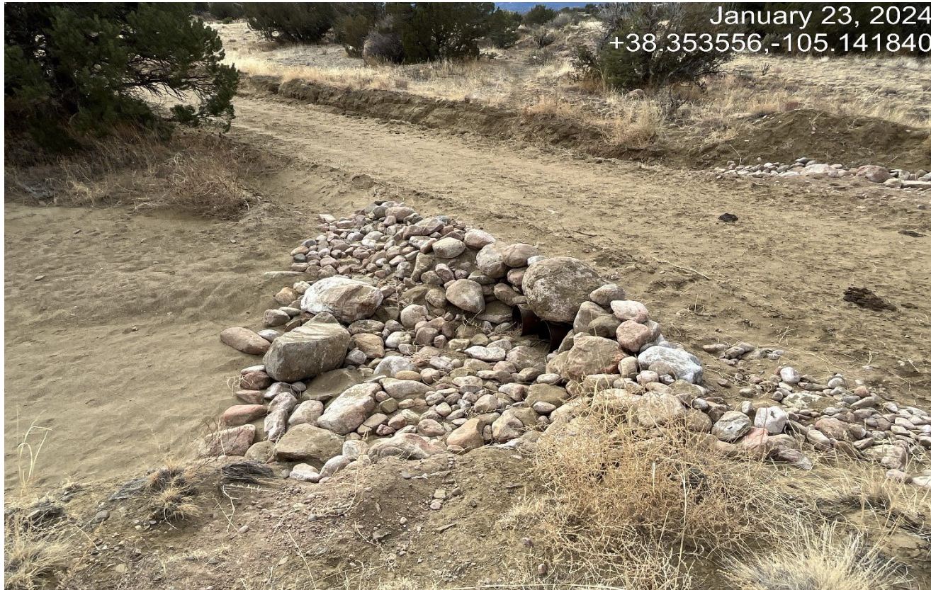
Photo 4. Facing toward the intermittent drainage that had washed out the road. There are two 1' culverts installed which may not be adequately sized for heavy storm events. The road rock used for outlet protection could become easily displaced.
