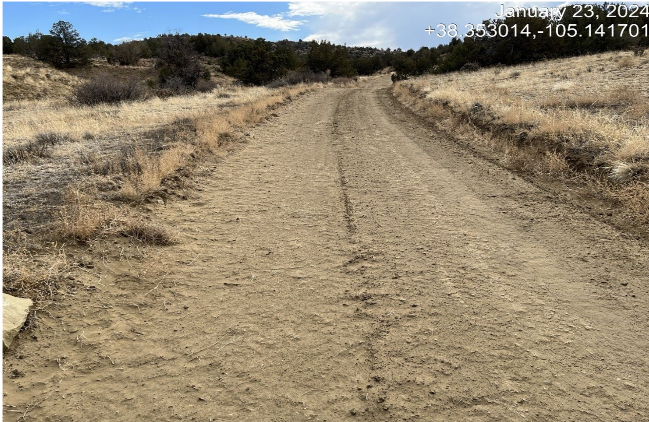
Photo 5. Further up along the access road facing southeast. The loose sandy soils are not stabilized and could easily erode.
