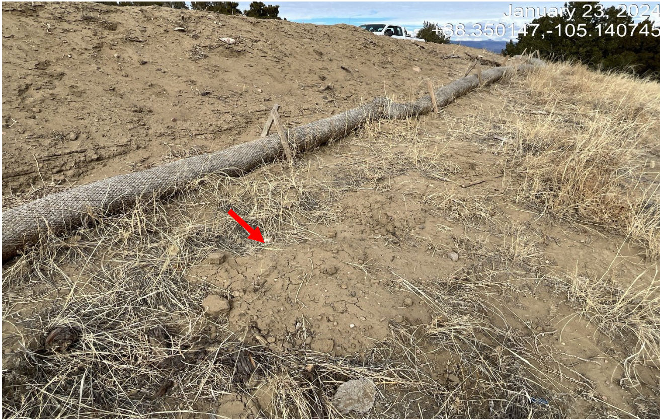
Photo 15. Facing along the east side of the location. It appears sediment along the wattles was cleaned out and shoveled toward the outside of the wattles shown at red arrow. The wattles are meant to contain sediment from leaving the site.
