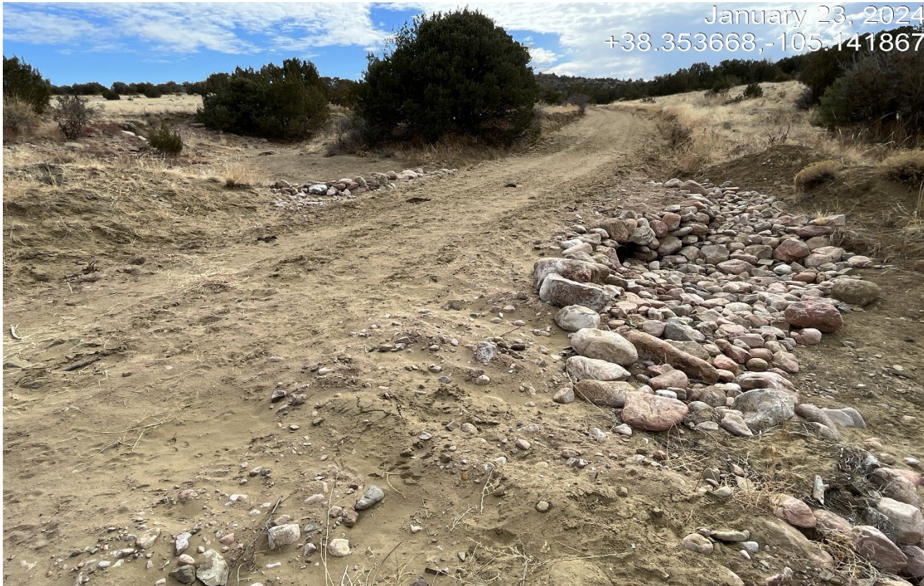
Photo 3. Facing toward the intermittent drainage that had washed out the road. There are two 1' culverts installed which may not be adequately sized for heavy storm events. The road rock used for outlet protection could become easily displaced.
