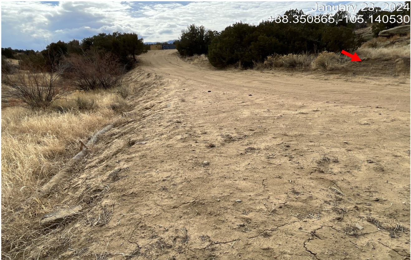
Photo 7. Facing south where soils were pushed out along the road side. Disturbed soils need to be replaced (at red arrow) and reclaimed.
