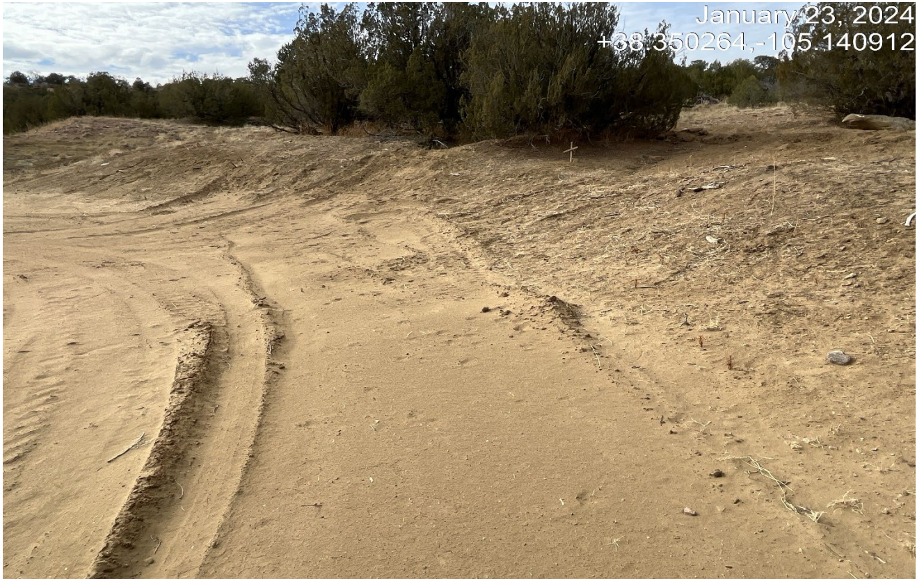
Photo 20. Facing southwest at the location. The cut slope of the location is not stabilized and there are insufficient stormwater run-on controls.
