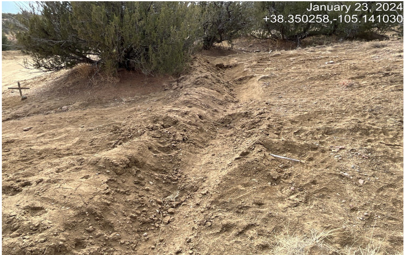
Photo 22. A small ditch was installed above the northwest side however, loose disturbed soils are susceptible to erosion.
