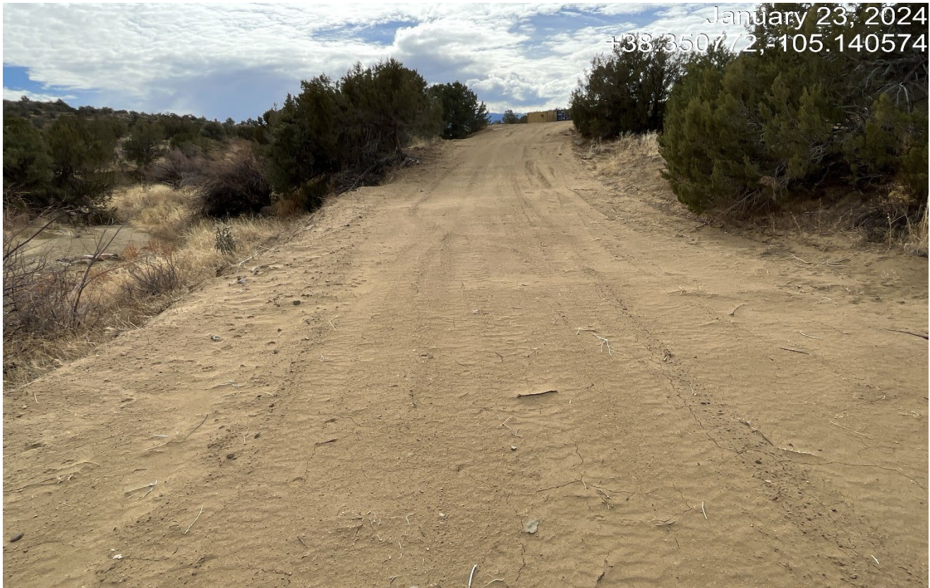
Photo 11. Facing south along the access road to the wellsite location. The erosion along this area was repaired however BMP's have not been installed and loose soils are susceptible to erosion.
