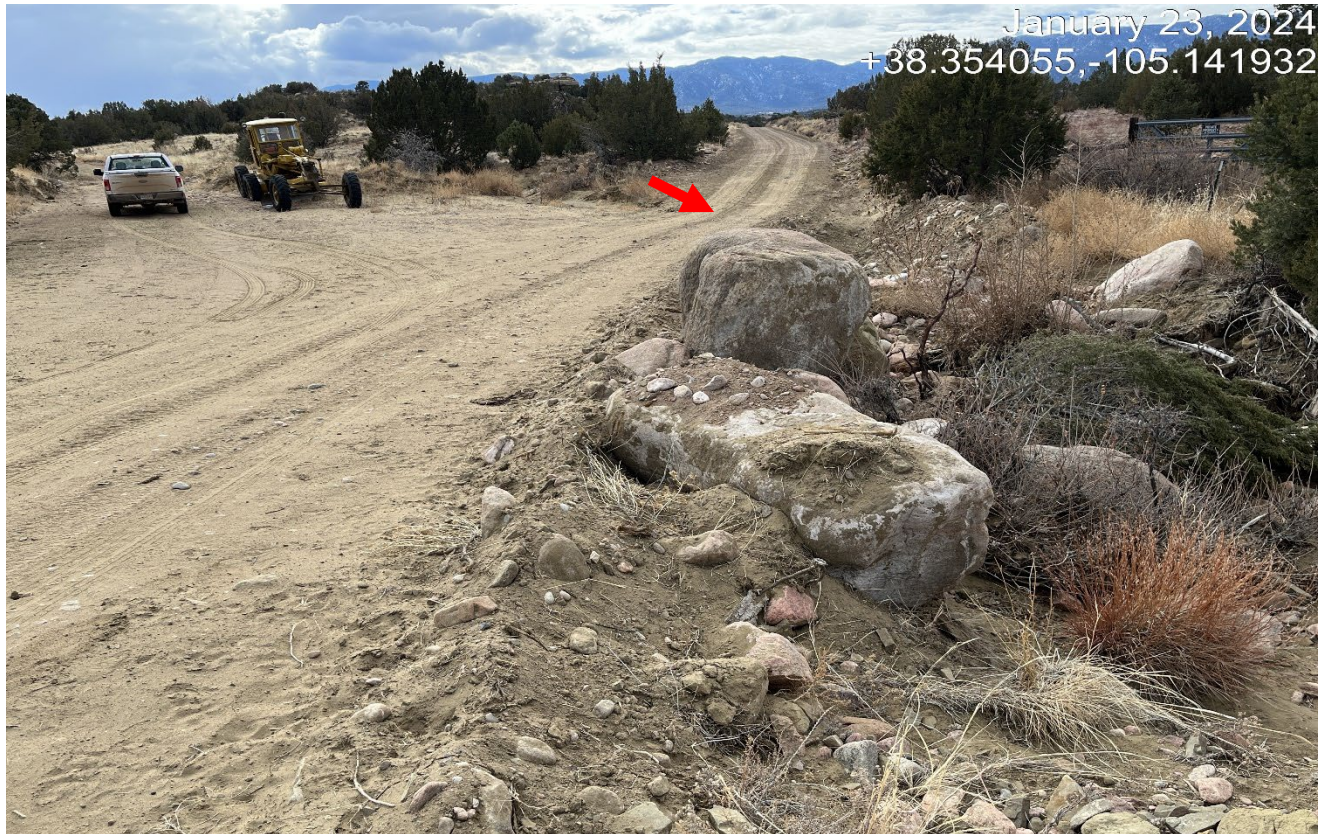
Photo 2. Facing south standing further back where the intermittent drainage crosses the road at red arrow. The rocks, sediment, and debris have been pushed out into the drainage at right side of the photo.
