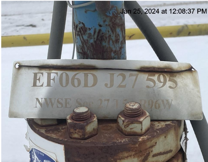
Photo # 3943 Wellhead signage insufficient/sign does not conform to CECMC rules
