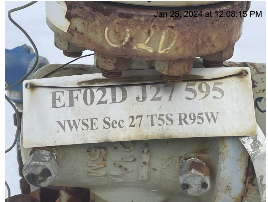
Photo # 3942 Wellhead signage insufficient/sign does not conform to CECMC rules
