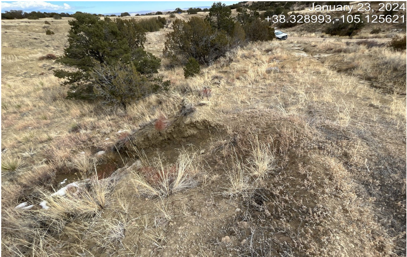
Photo 4. Further up along the access road facing northeast. There is an erosion channel directed down to the left side off the road.
