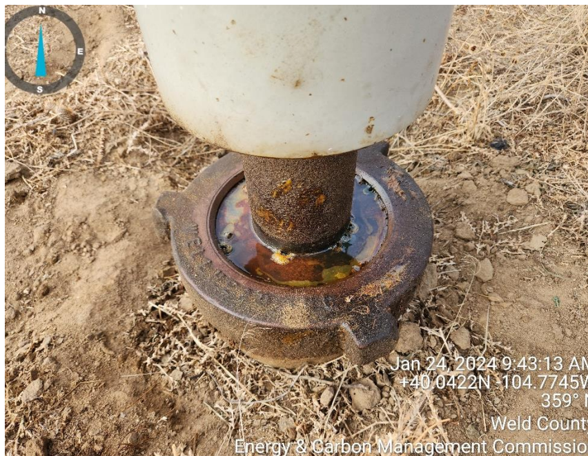
Photo 3 braden head leak
