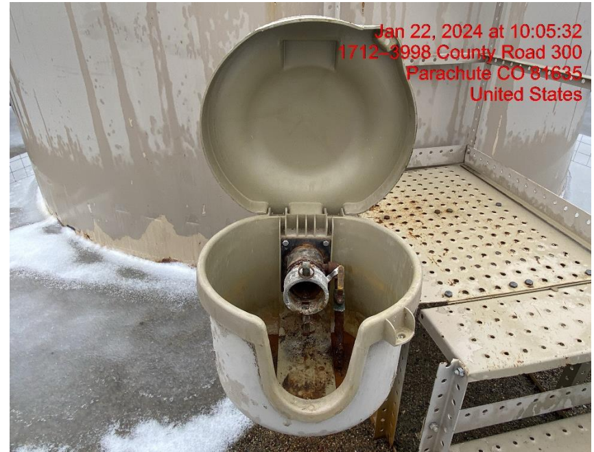
Open-Ended Load Line – Photo #08825
