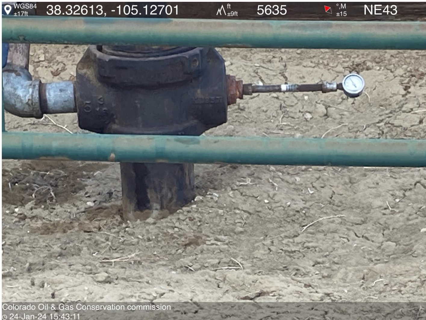
PHOTO 5: Bradenhead inaccessible or not visible( wellhead tree does not appear to include a Bradenhead in it original install). Install appropriate fittings to allow bradenhead visual inspection as per Rule 419.a.(1), (2). Ca date 1-31-2024.
