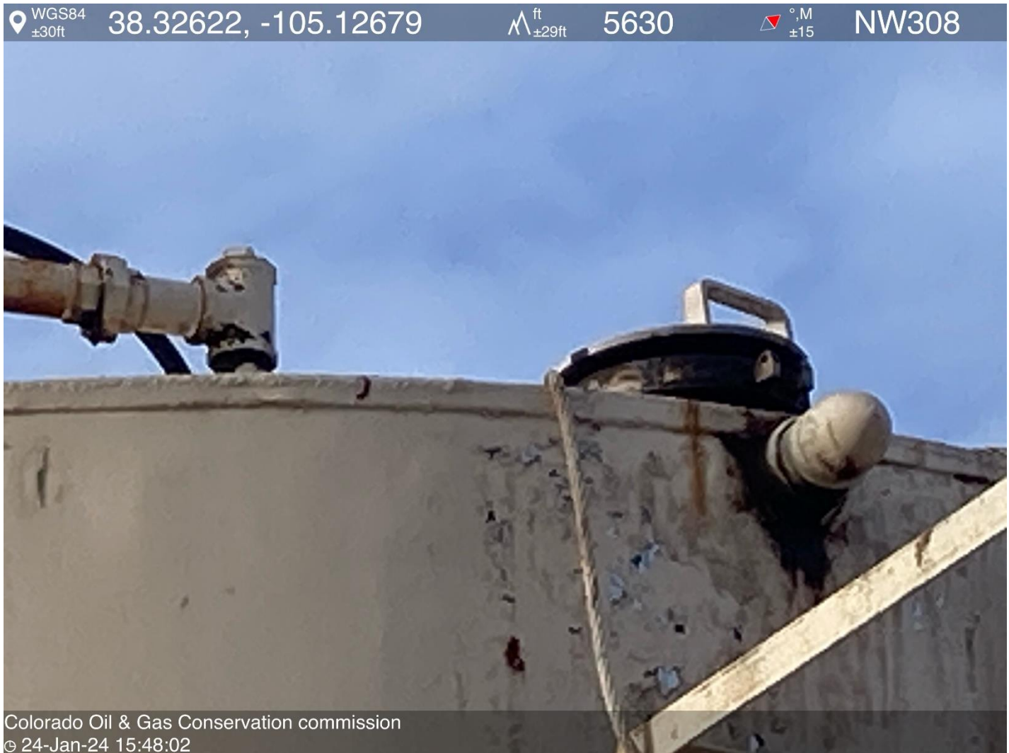
PHOTO 6: APPEARS THAT GUAGEHATCH LATCH IS BROKEN OR MISSING ON GUAGE HATCH AND THERE IS NO SAFETY VALVE INSTALLED ON TANK. Tanks will function as sealed and ventless with gas released only through a vapor control system or properly sized pressure relief valve. per Rule 608.a.(9). 24 HOURS TO INSTALL PRESSURE RELEIF VALVE. CA DATE 2-24-2024
