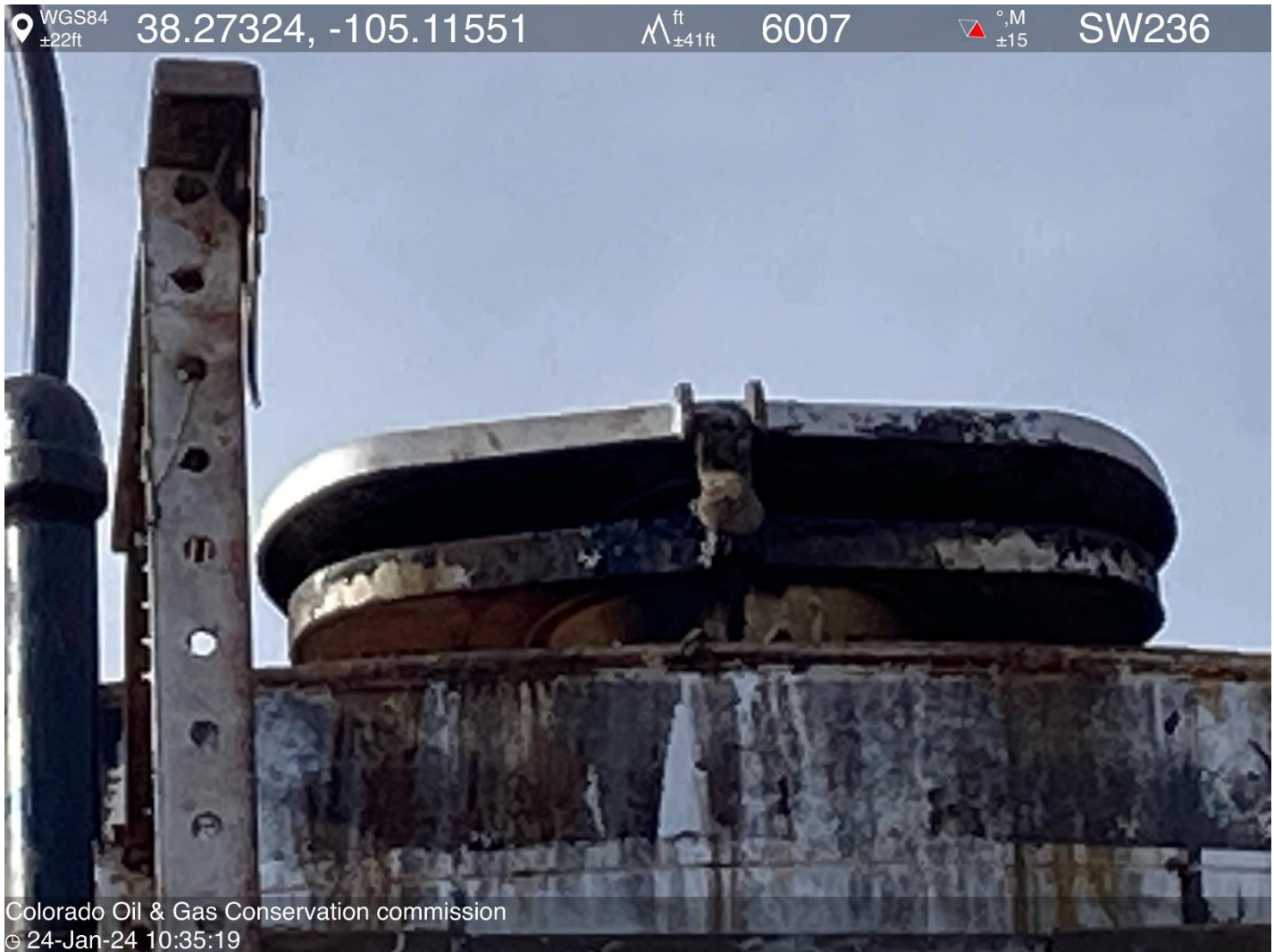
PHOTO 5: GAUGE HATCH IS NOT LATCHED. Close and seal gauge hatches when not accessing tank per Rule 608.a.(9). 24 HOURS TO ADDRESS. Tanks will function as sealed and ventless with gas released only through a vapor control system or properly sized pressure relief valve. per Rule 608.a.(9). 24 HOURS TO INSTALL PRESSURE RELIEF VALVE. THIS IS THE SECOND NOTICE IMMEDIATE ACTION IS REQUIRED.
