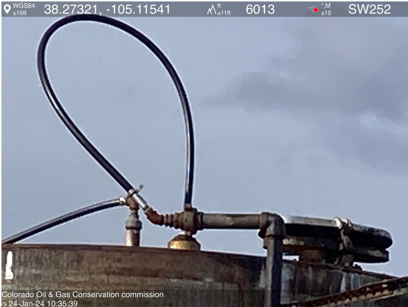
PHOTO 6: NO PRESSURE RELIEF VALVE INSTALLED ON CRUDE OIL TANK. Close and seal gauge hatches when not accessing tank per Rule 608.a.(9). 24 HOURS TO ADDRESS. Tanks will function as sealed and ventless with gas released only through a vapor control system or properly sized pressure relief valve. per Rule 608.a.(9). 24 HOURS TO INSTALL PRESSURE RELIEF VALVE. THIS IS THE SECOND NOTICE IMMEDIATE ACTION IS REQUIRED.
