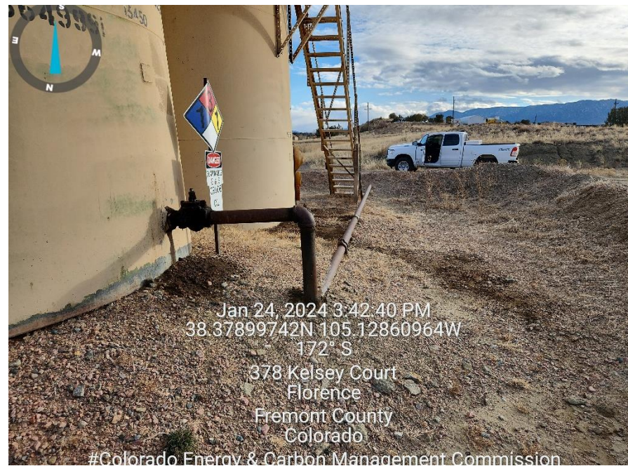
Photo 4 Stained soil and mechanical issue crude oil load lines.
