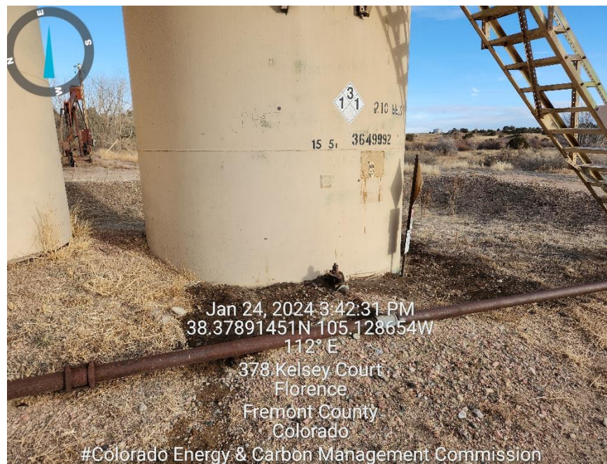
Photo 3 Stained soil and mechanical issue crude oil load lines.
