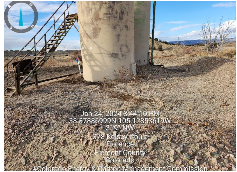
Photo 8 Stained soil and mechanical issue crude oil load lines.
