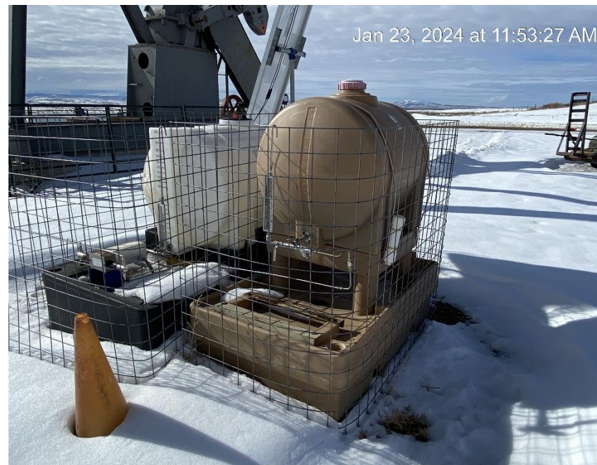
Chemical tanks lacking required labels
