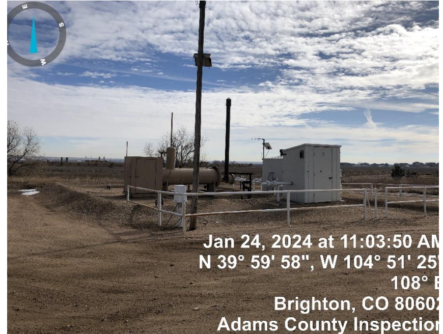
Photo#2 Separator/ECD/(2) Gas Meters
