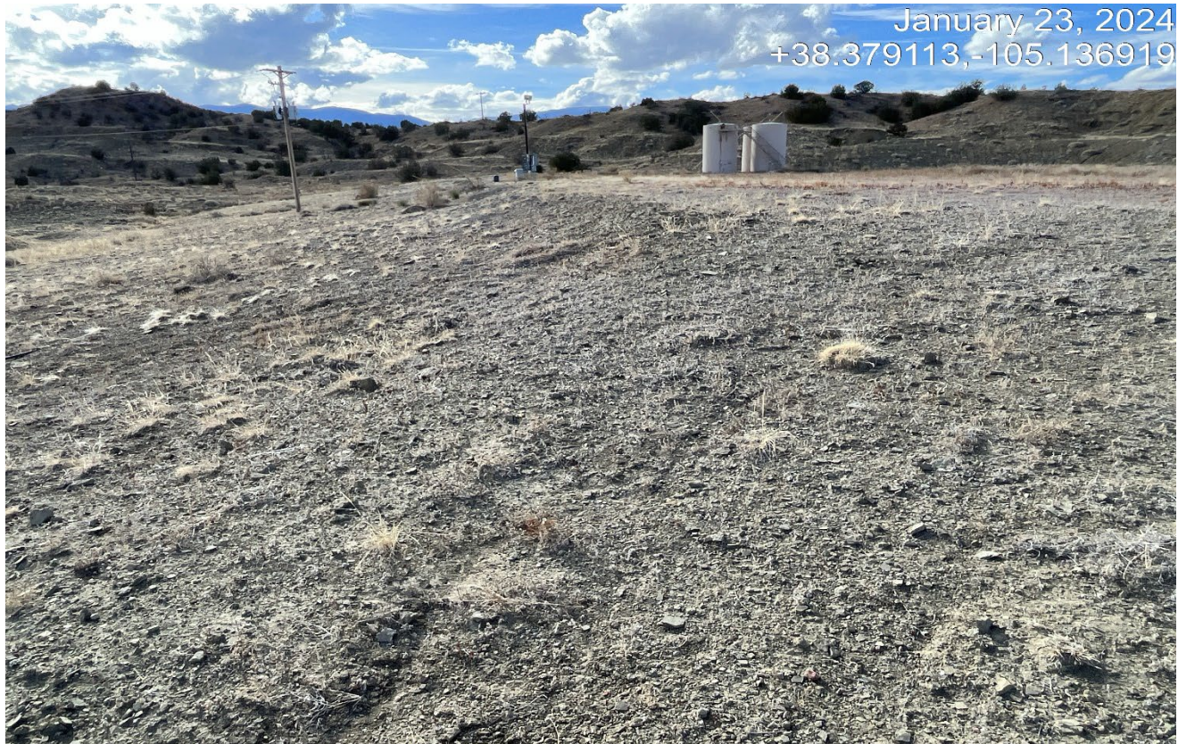
Photo 4. Facing southwest along the fill slope. The location will need to be recontoured back to the original slopes
