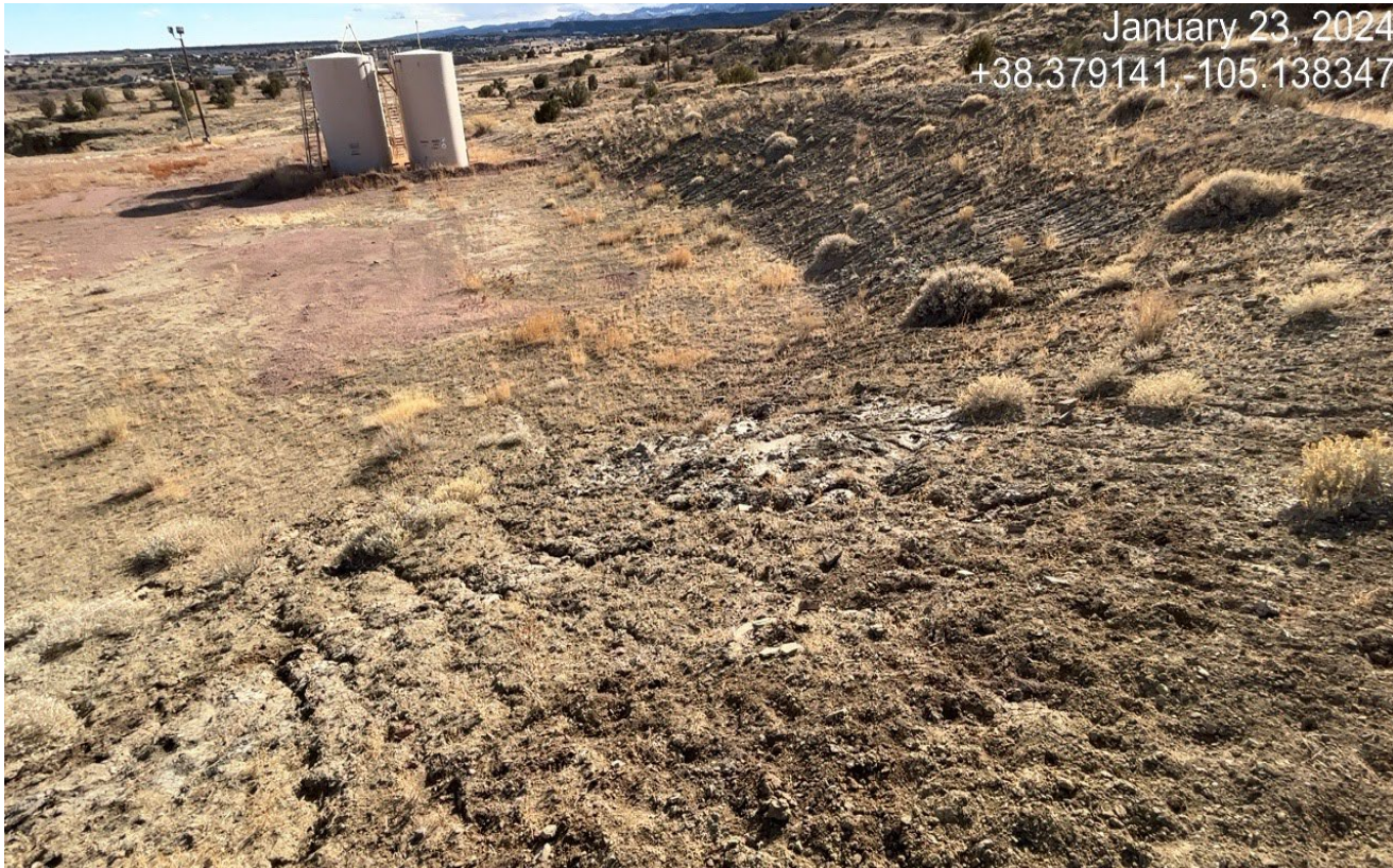
Photo 10. Facing east along the cut slope. There is rilling erosion along the cut slope.
