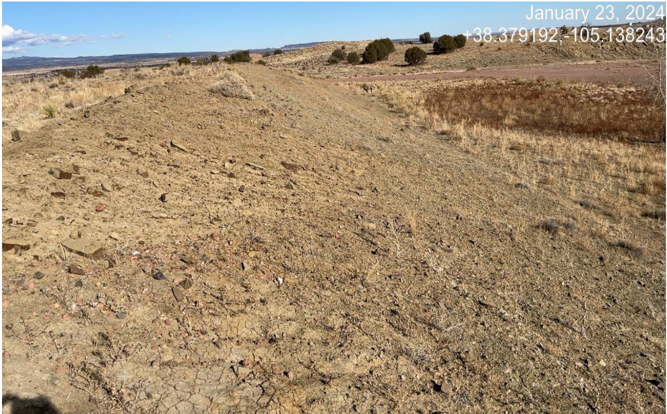
Photo 11. Facing north along the cut slope. There cut slope is not stabilized.
