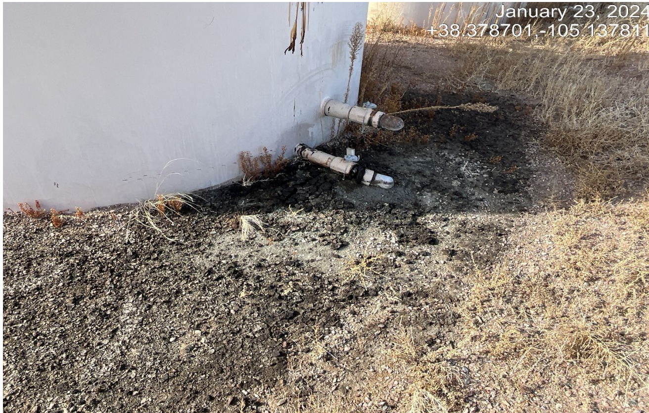
Photo 7. Upon closer inspection of the tanks there is a spill that had occurred at the tank outlet. Immediate clean up needs to be performed.
