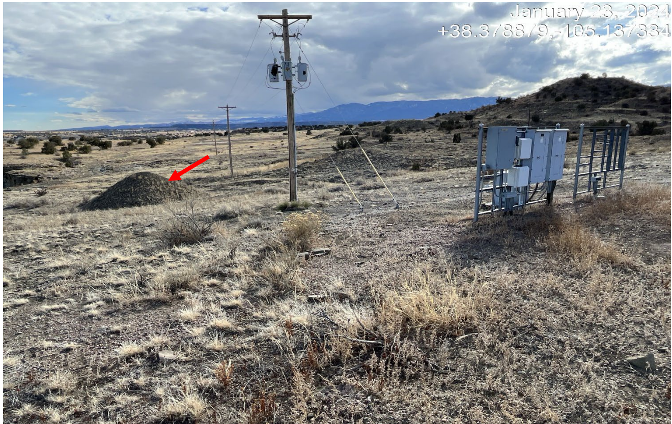
Photo 5. The electric utilities remain at the location and should have been removed with 3 months of abandonment. The entire powerline and poles servicing this location must be removed. There is a topsoil pile shown at red arrow.
