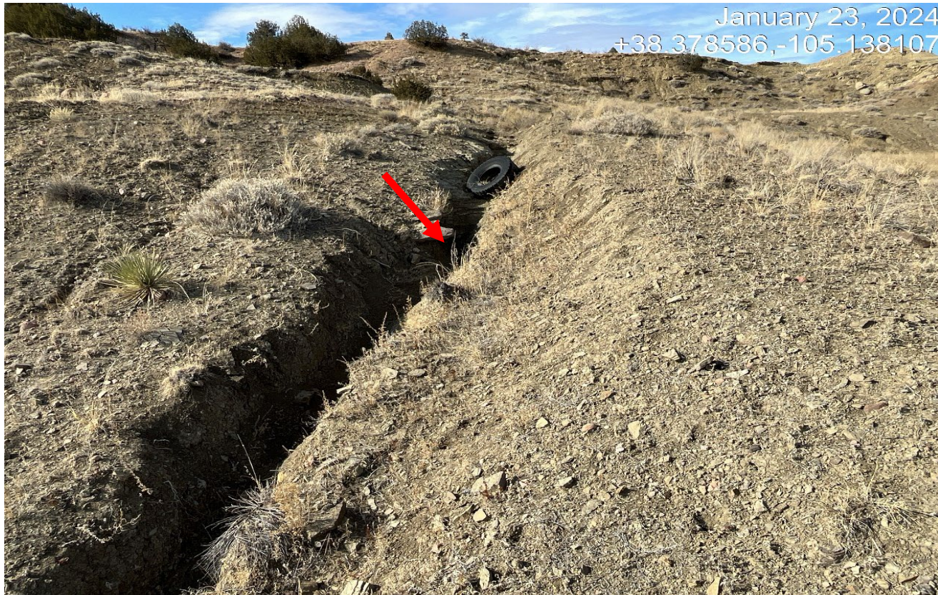
Photo 8. Facing west at the south side of the location. There is an erosion channel shown at red arrow which will need to be repaired and stabilized.
