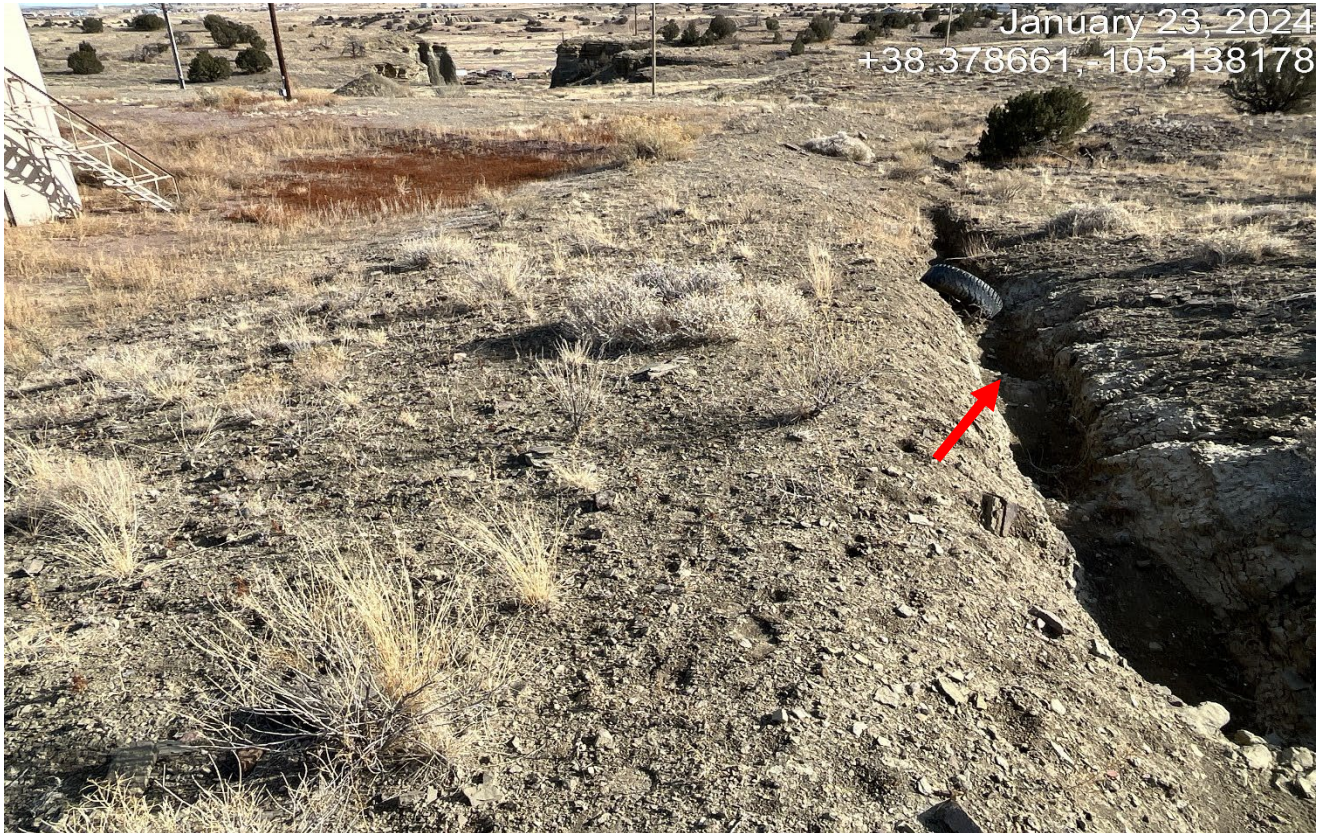
Photo 9. Facing southeast at the south side of the location. There is an erosion channel shown at red arrow which will need to be repaired and stabilized.
