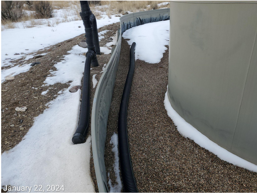
Photo 3: Unused pipe stored within the battery facility's containment BMP.
