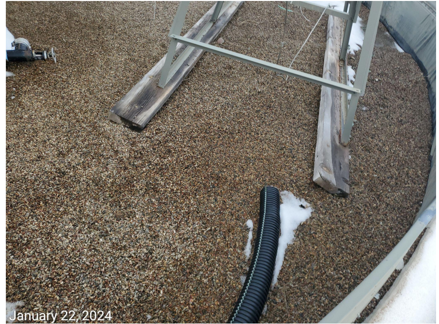
Photo 3: Unused pipe stored within the battery facility's containment BMP.
