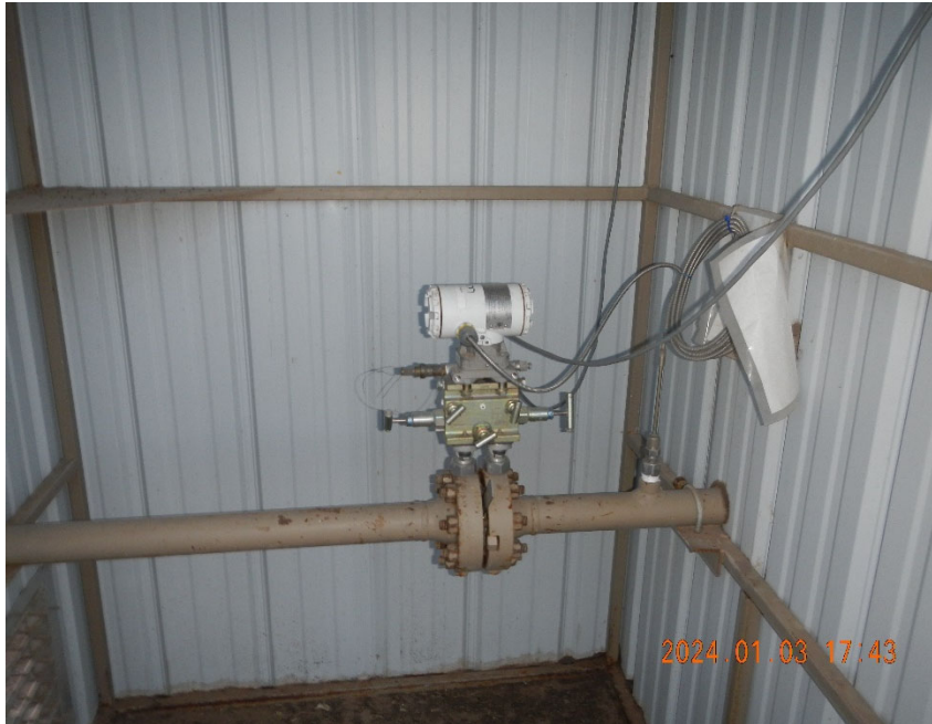
7. Digital gas meter inside meter shed.
