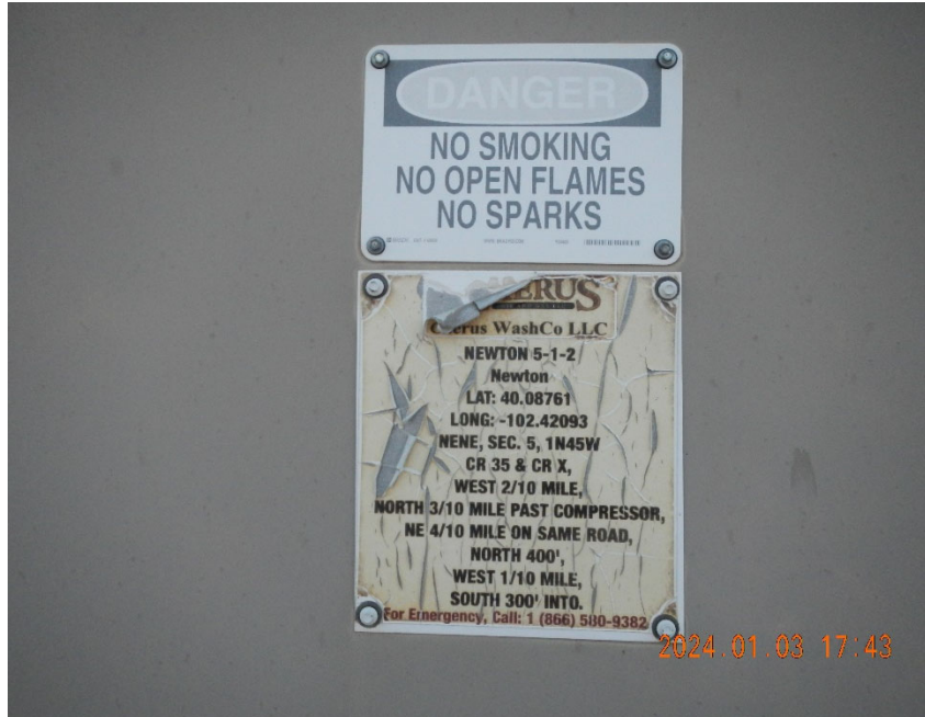
5. Well sign on remote meter shed door. Note incorrect operator and Emergency Contact Number.
