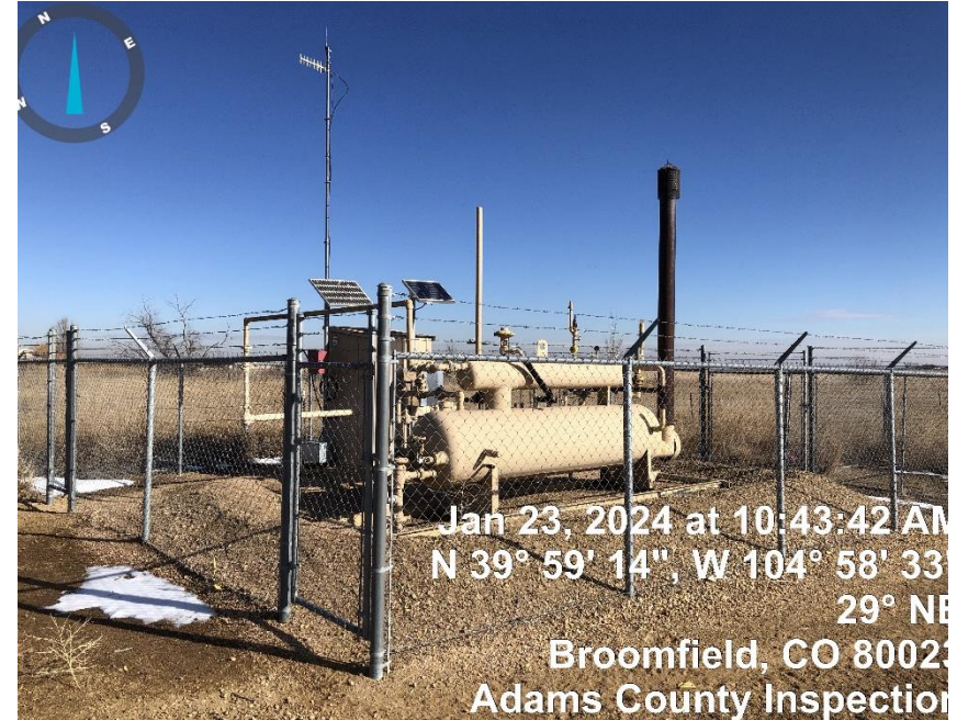
Photo#2 Separator/Gas Meter/Automation RTU
