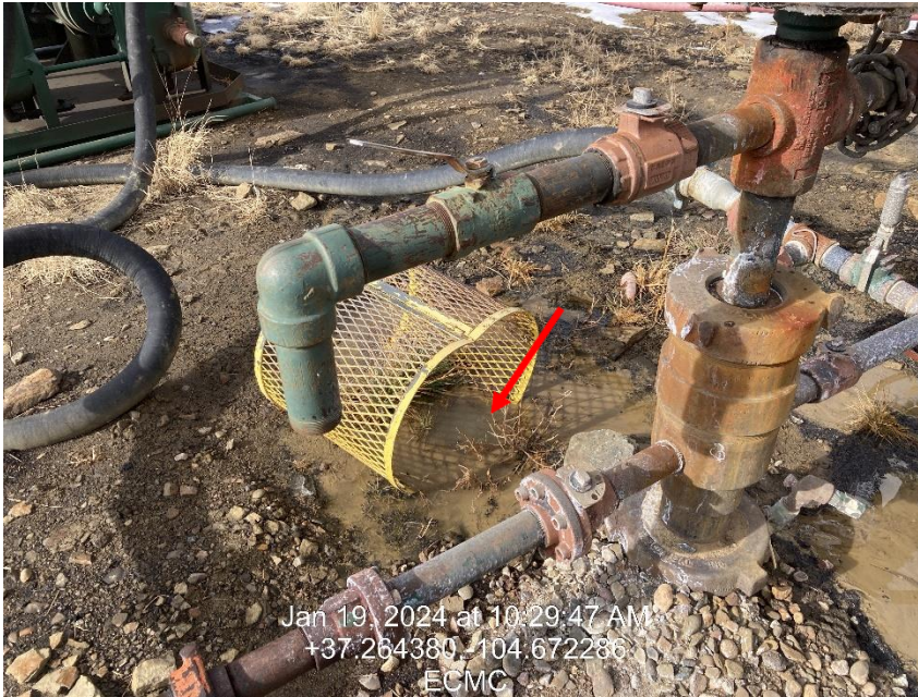
Photo 3 – Spill at wellhead
