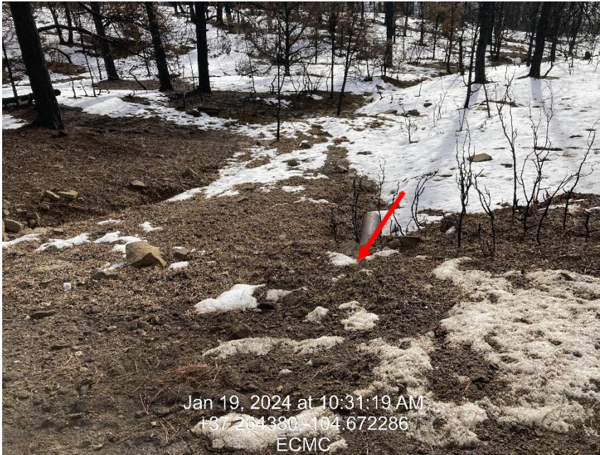
Photo 5 – Open End of Plugged Culvert at Lat 37.26438; Long -104.67228
