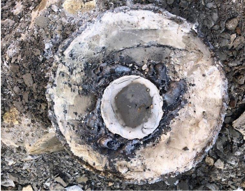
Cement to surface.
