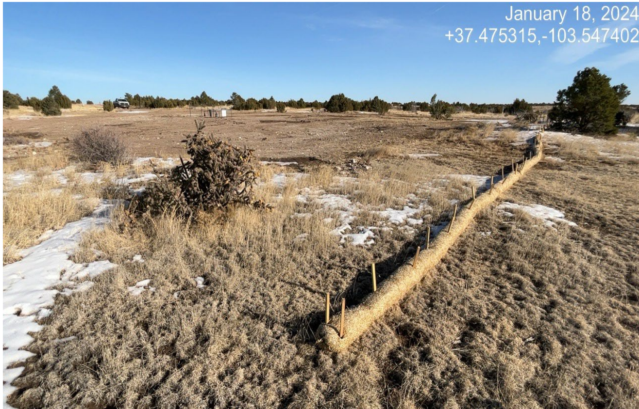
Photo 9. Facing southeast at the west side of the location. The perimeter wattles end at this point and do not protect the northwest downhill perimeter where loose soil are present.
