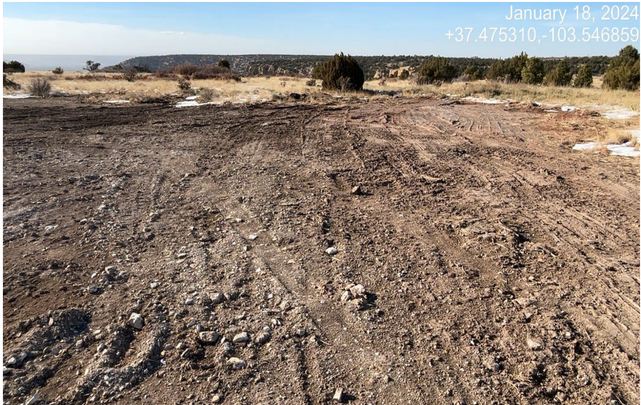
Photo 5. Facing northwest at the location where cuttings were improperly stored. It appears most of the drill cuttings have been removed. There are still no stormwater controls present at the northwest downslope side of the location.
