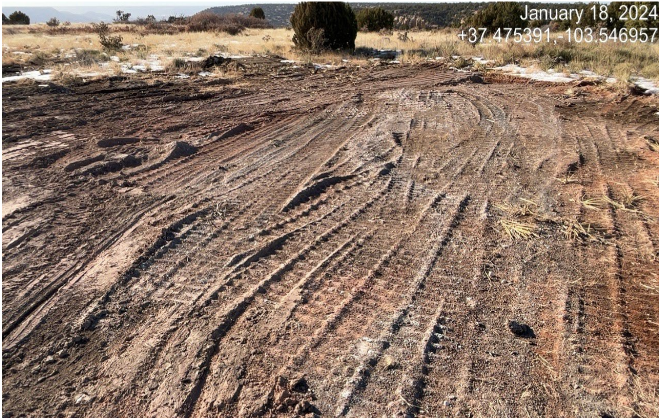
Photo 6. Facing toward the northwest side of the location. There is still a reddish color in this area that remains which is indicative of the drill cuttings.
