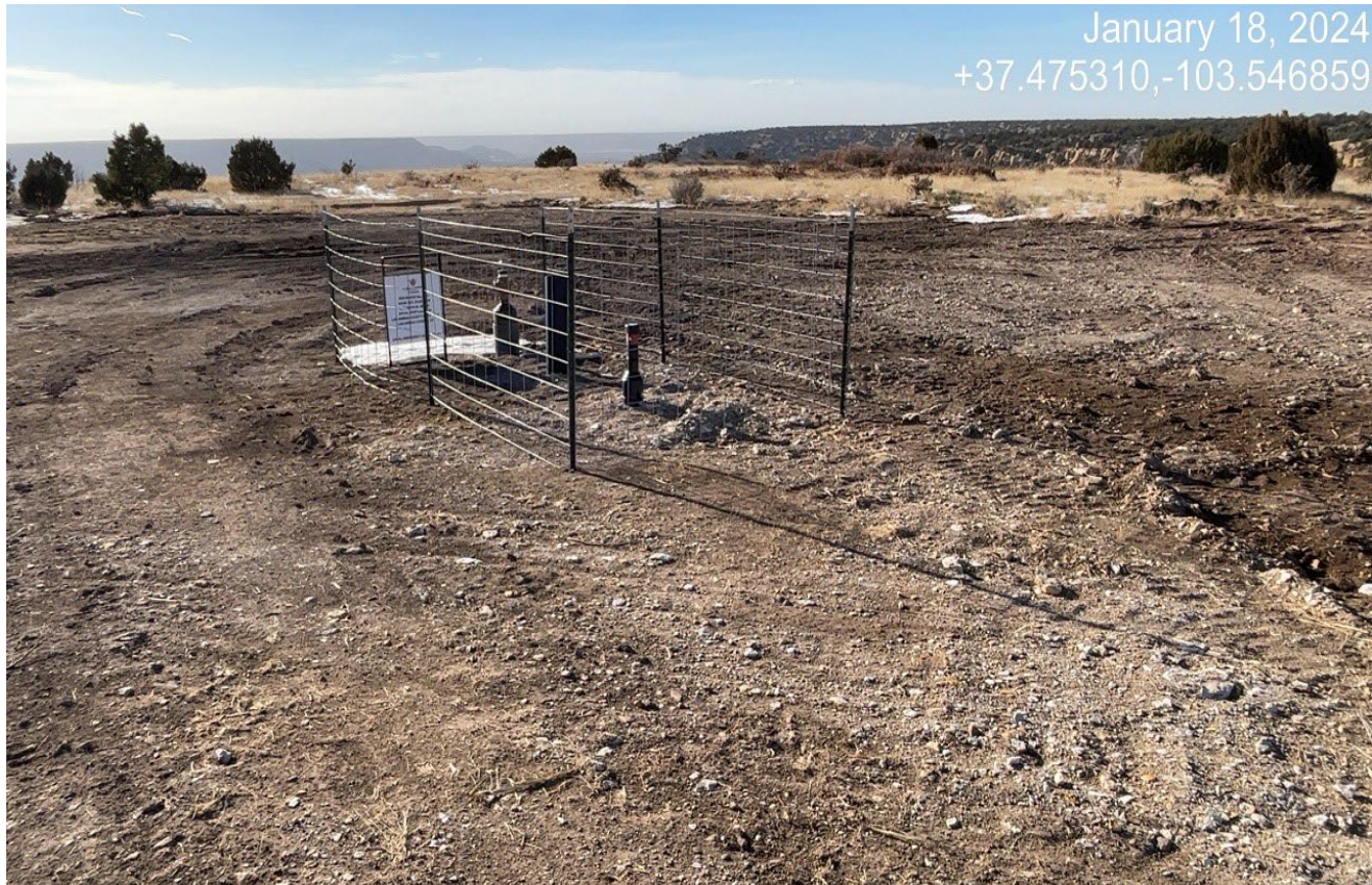
Photo 4. Facing toward the well. The excavated area near the well has been backfilled. Most of the rock debris has been removed. It is unknown what topsoil material was replaced since it was not properly salvaged.
