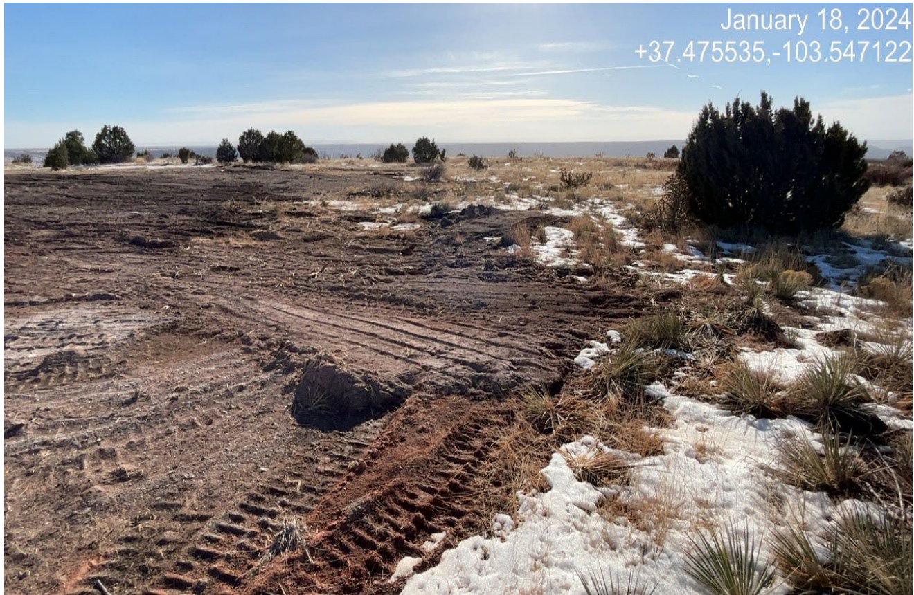
Photo 8. Facing southwest at the northwest side of the location. There are still no stormwater controls present at the northwest downslope side of the location. Previous corrective action has not been completed.
