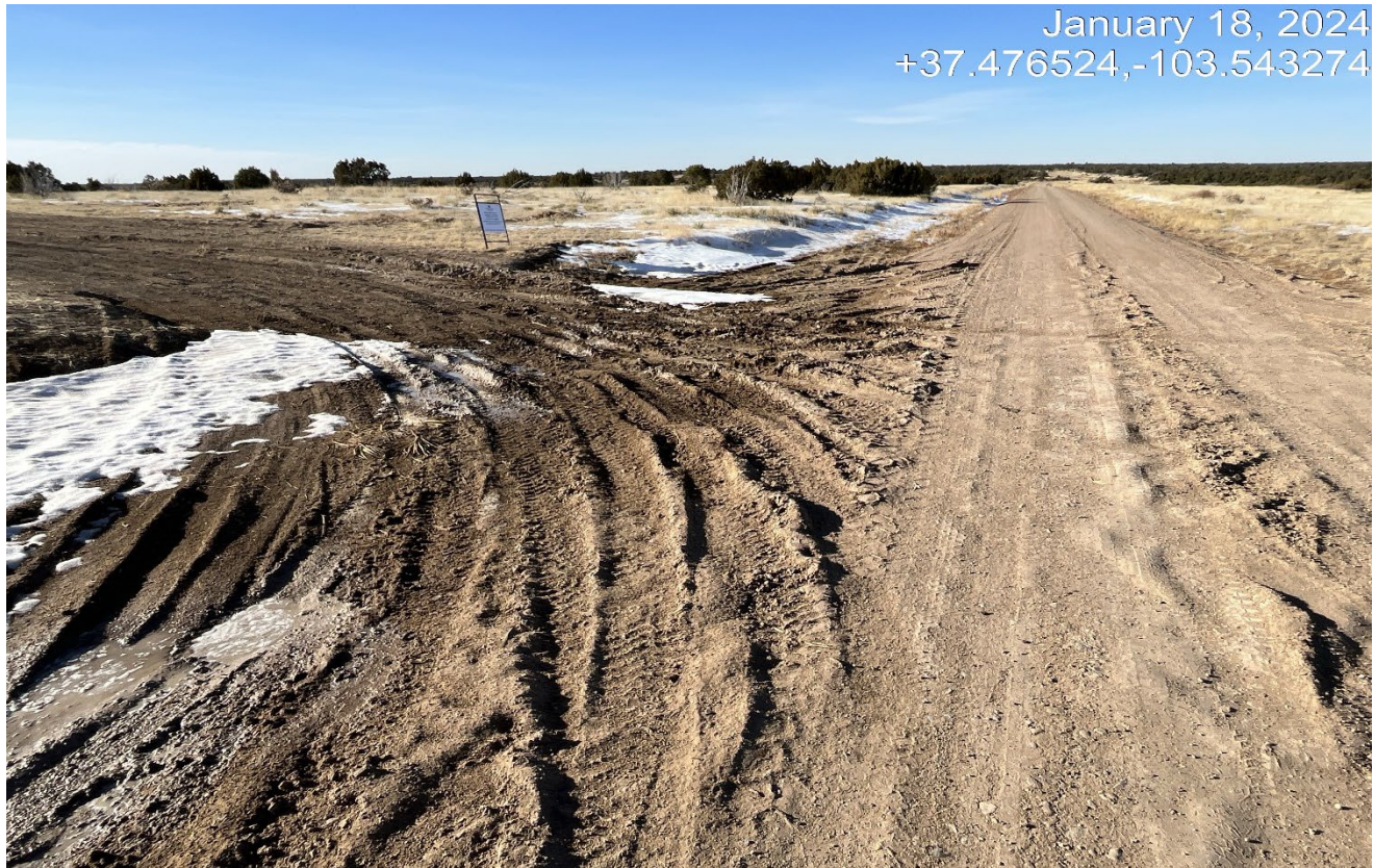
Photo 1. Facing northwest toward the access road and County Road 177. There is vehicle rutting and tracking of sediment onto the County Road. BMP's must installed to prevent sediment tracking and road degradation.
