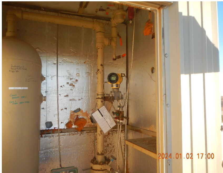
5. Digital gas meter inside meter shed.
