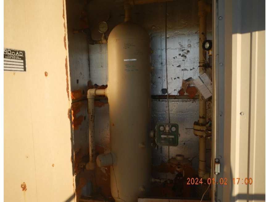
4. Vertical separator inside meter shed.
