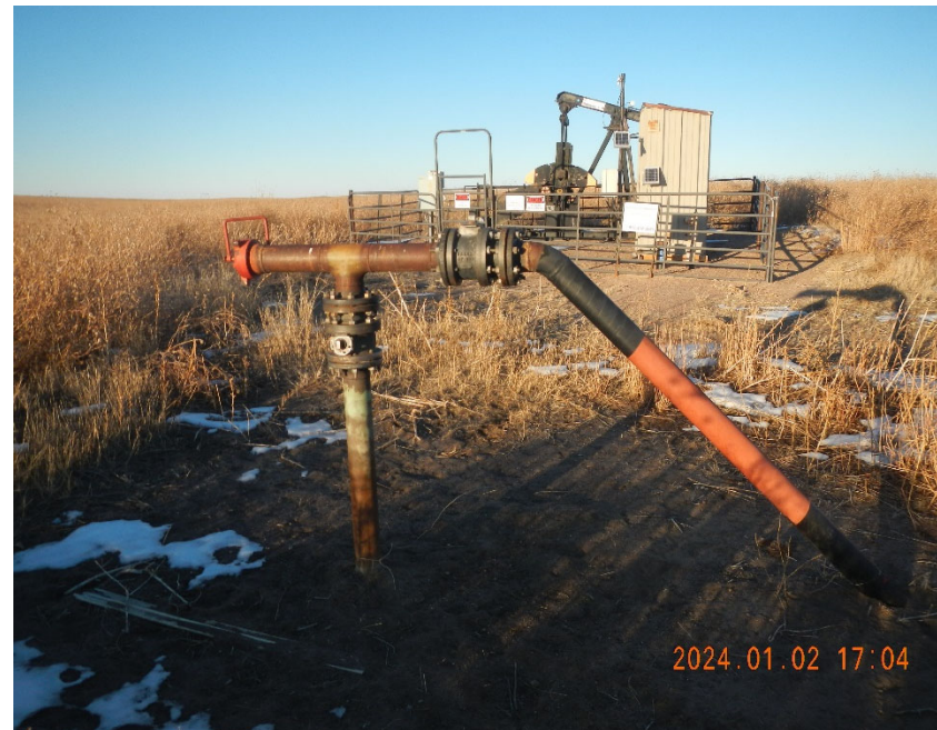
6. Pig station at location.
