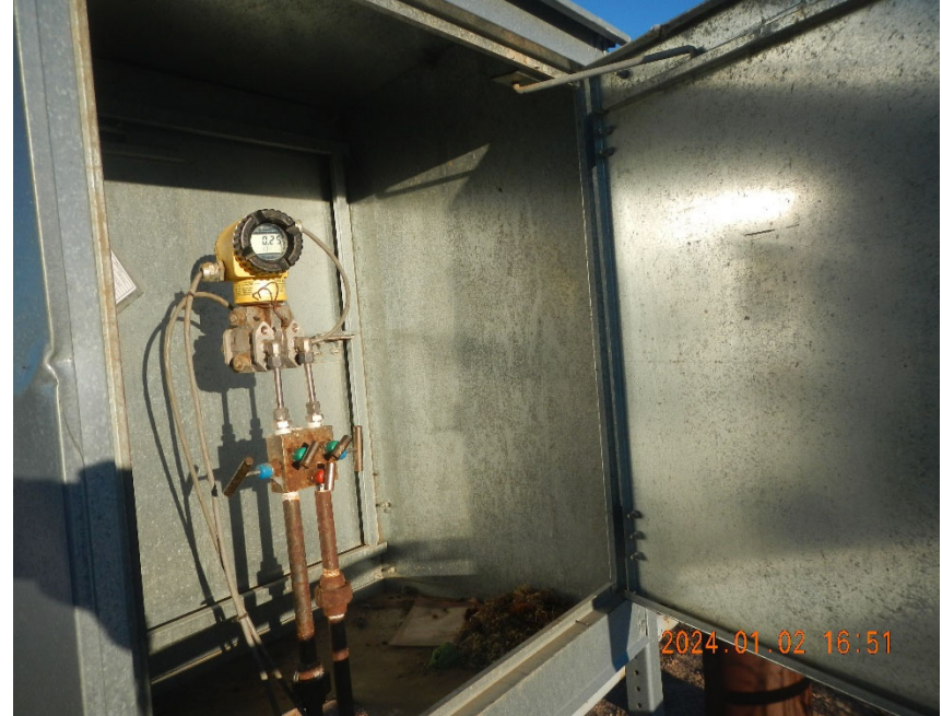
4. Digital gas meter inside meter box.
