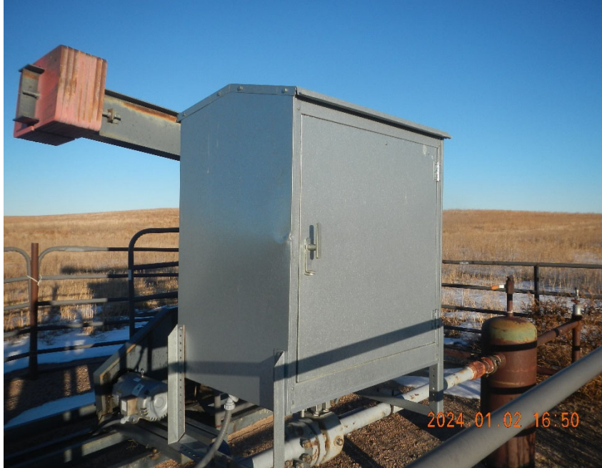
3. View of meter box mounted over flowline.
