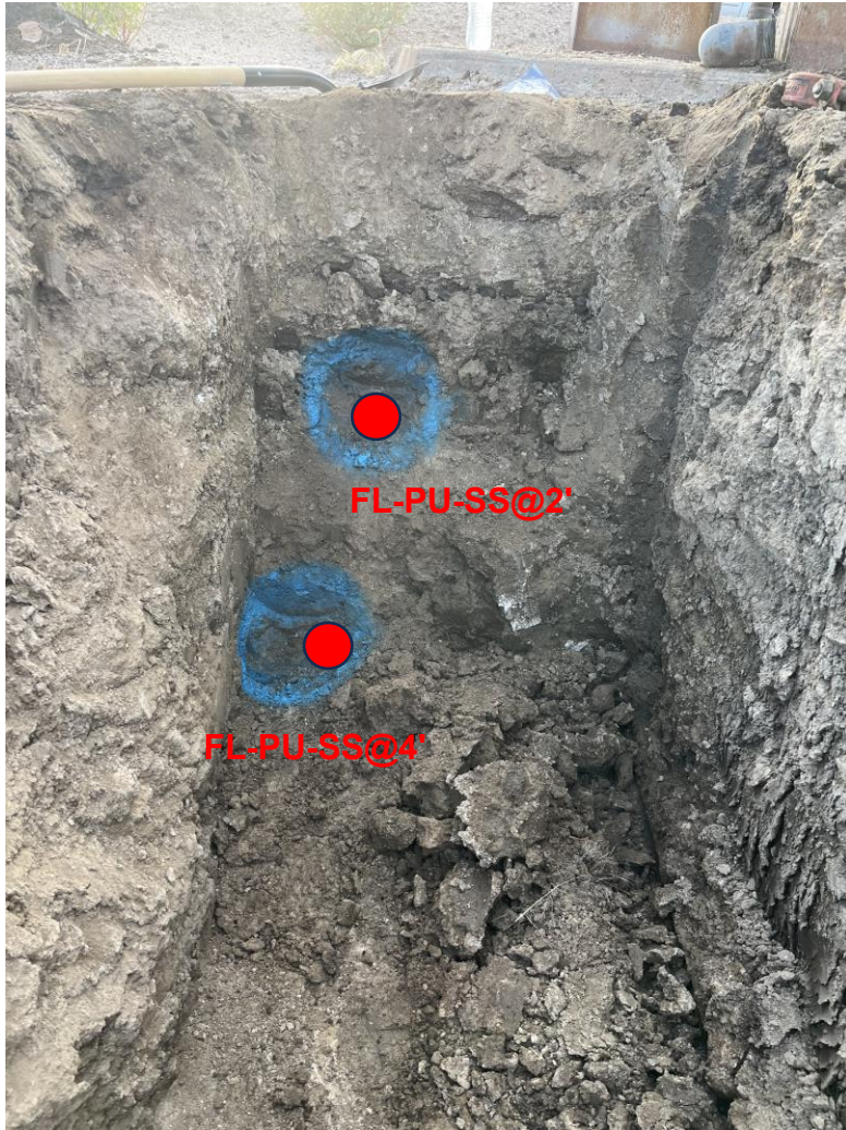
Flow Line End Point at Production unit. Flow line portion was Fiberglass and removed
