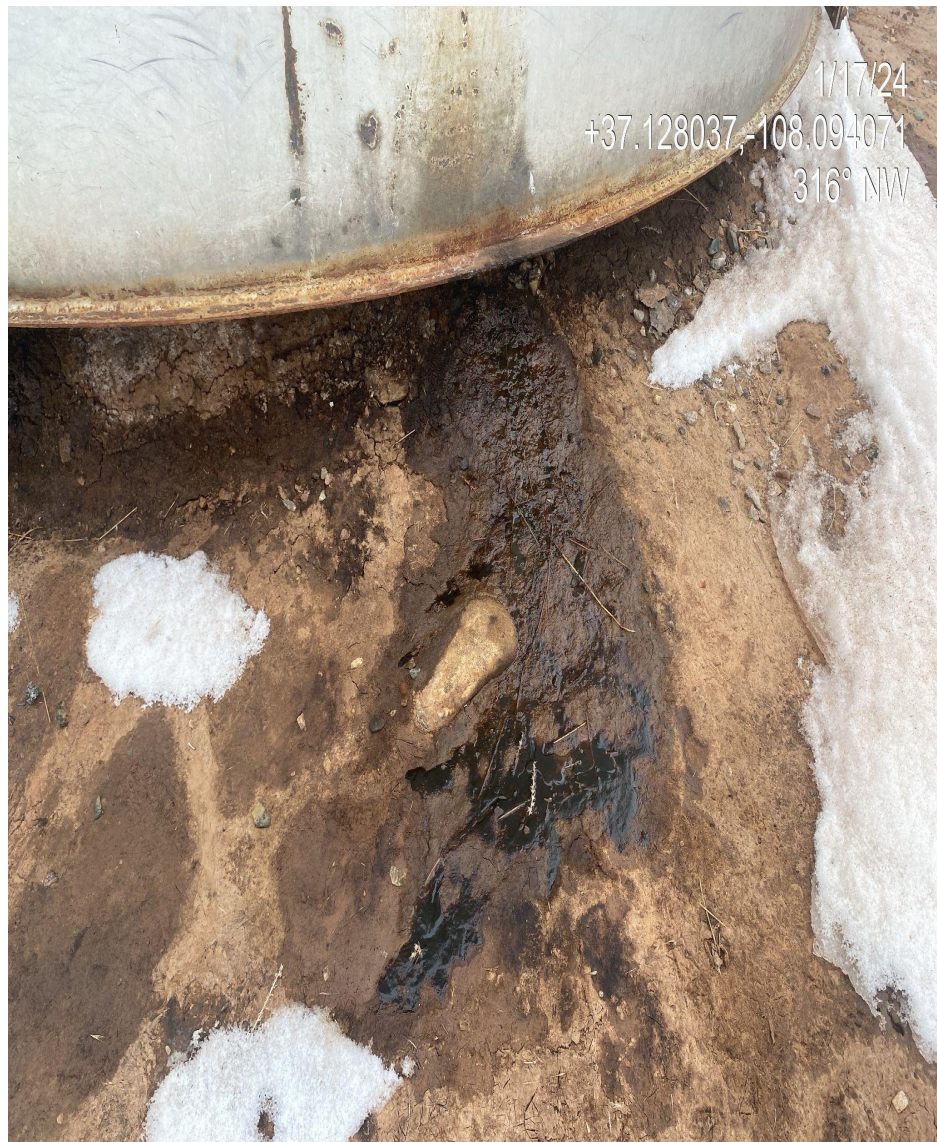
Photo 4. View of oily substance spilling from tank battery equipment.
