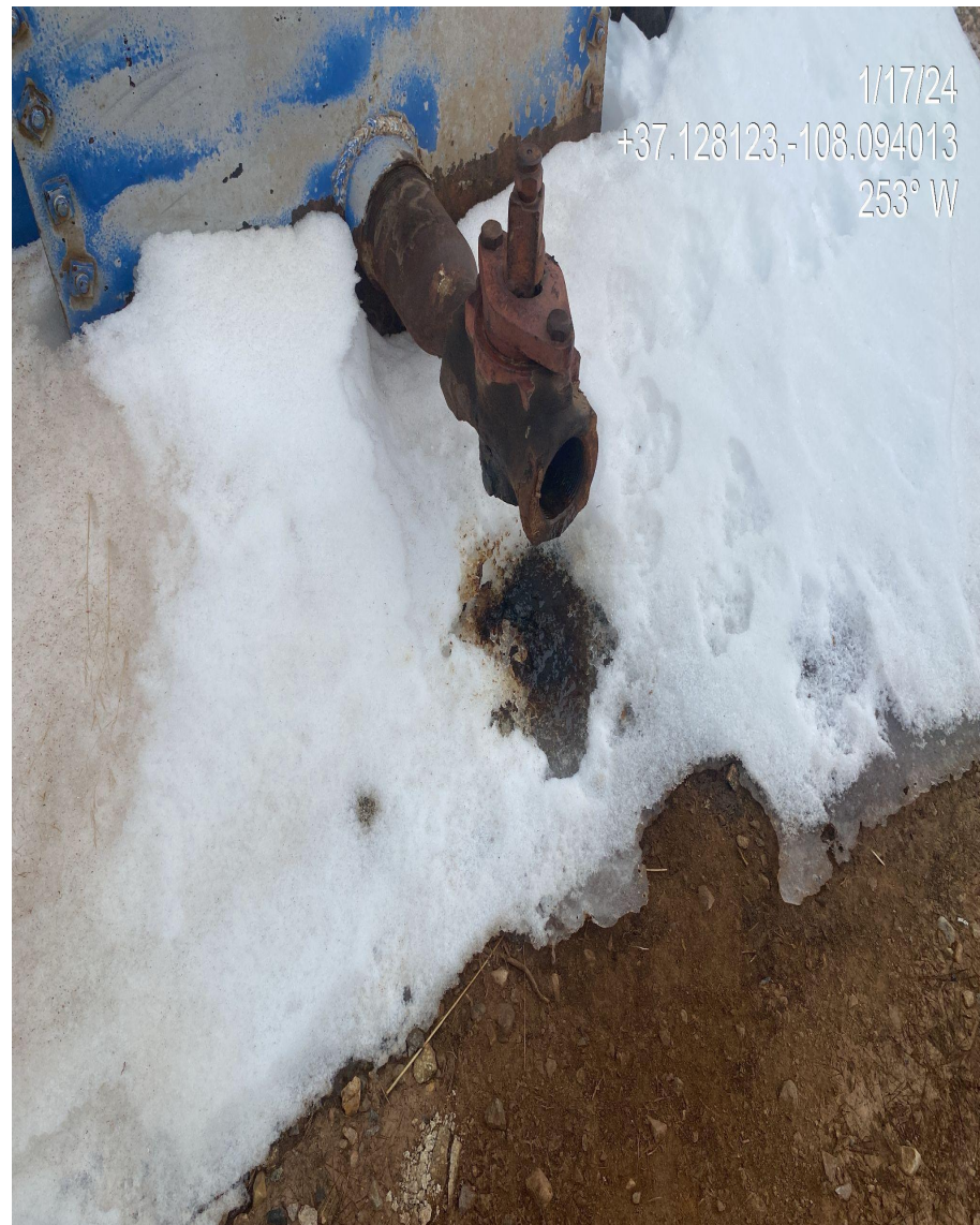
Photo 4. View of oily substance spilling from tank battery equipment.
