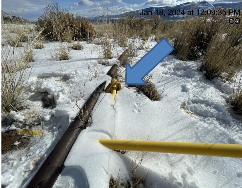
Photo # 3185 Improperly marked deadman
