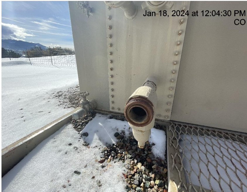
Photo # 3183 Open ended pipping on separator unit/wildlife hazard
