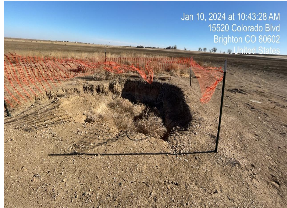
Photo 8. Photo of open excavation filled with weed debris and inadequate fencing. Photo taken facing east.
