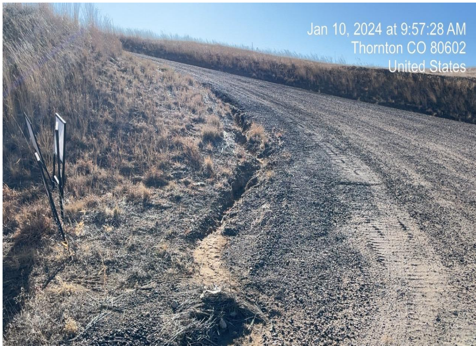
Photo 3. Photo taken of stormwater erosion at entrance of pad. Photo taken facing south.
