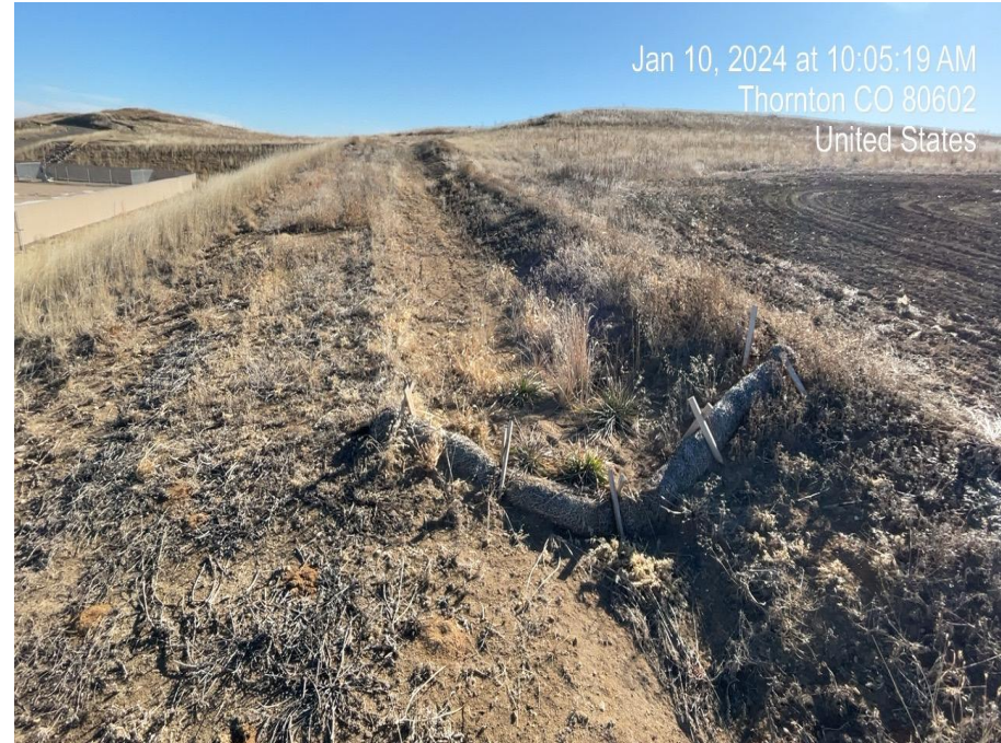
Photo 6. Photo of sediment filled wattle check dam in drainage on south side of location. . Photo taken facing east
