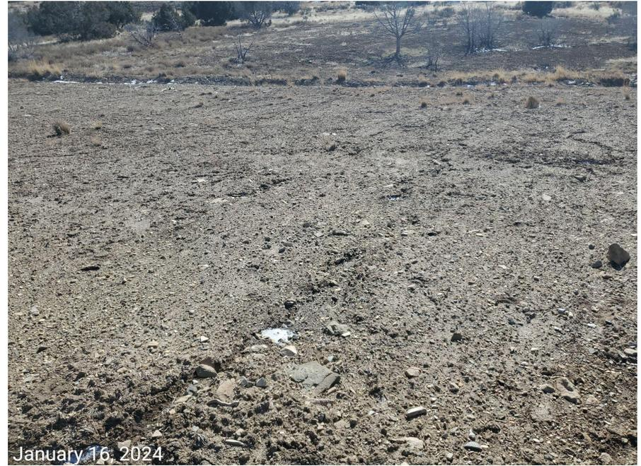
**Photo 4:** Photos taken from the western interim areas of the Location. Areas are predominantly bare and exposed soils. Little to no desirable vegetative establishment is occurring in these areas. BMPs to minimize erosion, degradation and sediment transport also missing or insufficient; rill erosion observed.
