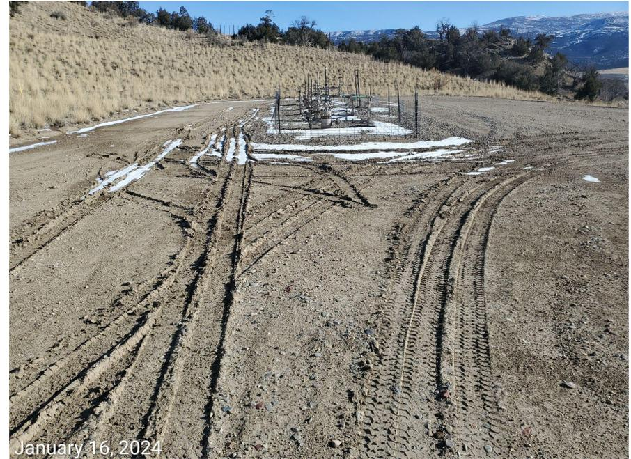
**Photo 5:** Photos taken from the working pad surface around the wells. Photos examples showing BMPs to stabilize the working pad surface are no longer in proper functioning condition; control measures to minimize tracking inadequate; control measures to minimize off-site sediment transport by equipment, such as vehicle tracking pad, also not observed.
