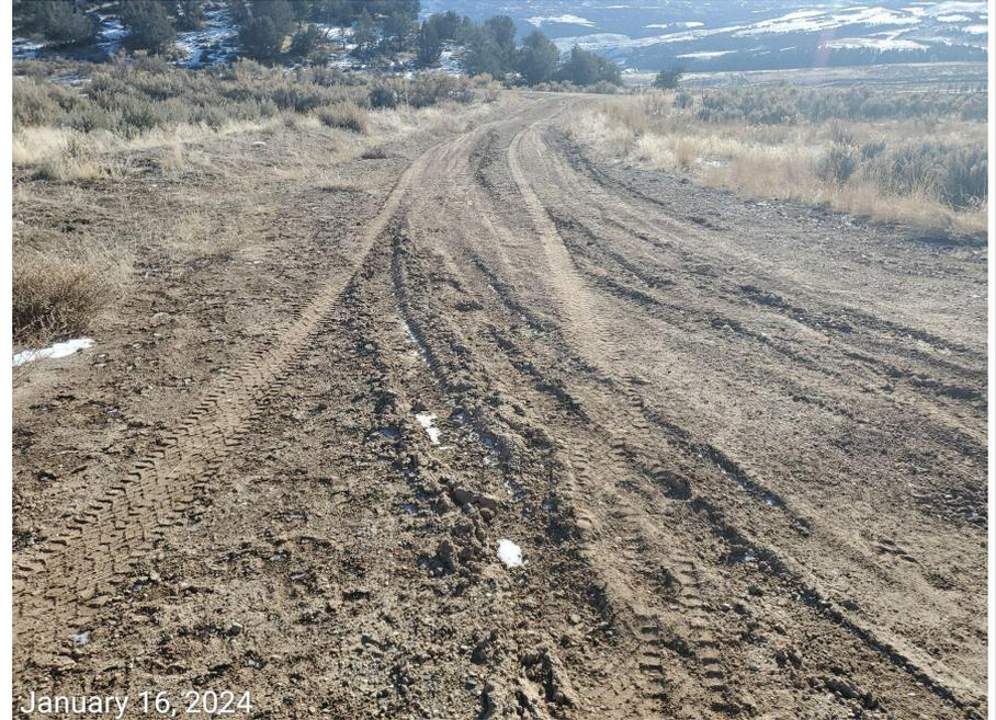
**Photo 3:** Photos examples showing BMPs to stabilize the working pad surface and access road are not longer in proper functioning condition; control measures to minimize tracking inadequate; control measures to minimize off-site sediment transport by equipment, such as a vehicle tracking pad, also not observed.
