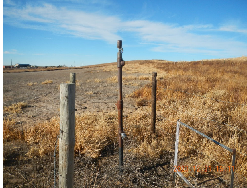
6. Additional view of Flowline riser open at T connection.
