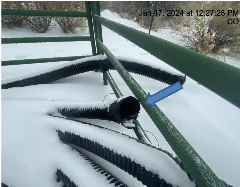
Photo # 3004 Flowline heating insulation open ended/wildlife hazard
