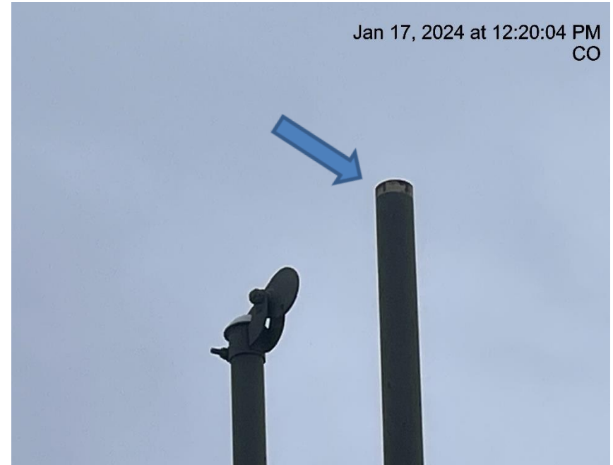
Photo # 3007 Rupture disc vent line lacks cap
