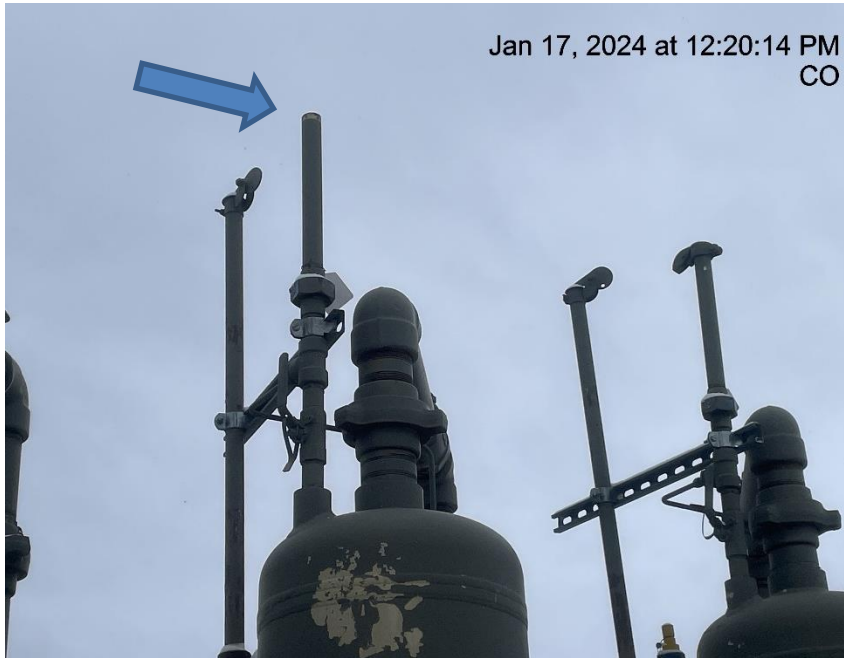
Photo # 3006 Rupture disc vent line lacks cap
