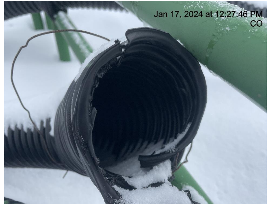
Photo # 3005 Flowline heating insulation open ended/wildlife hazard
