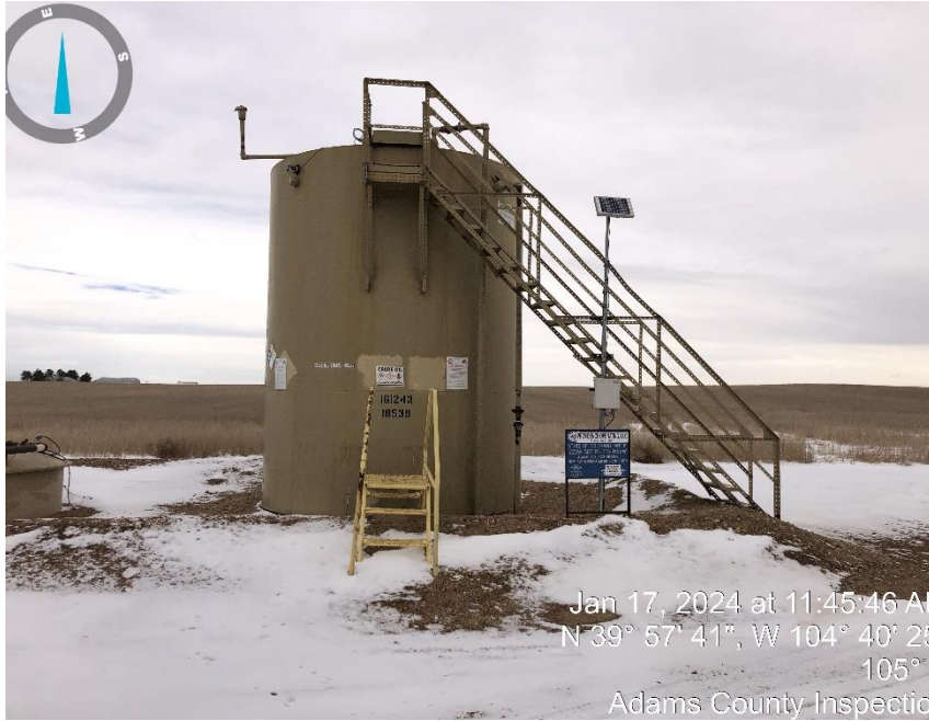
Photo #1 Crude tank.
