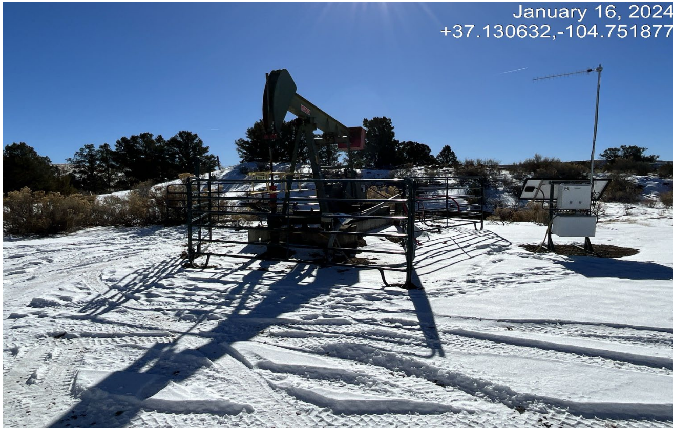
Photo 2. Facing south at the wellsite.
