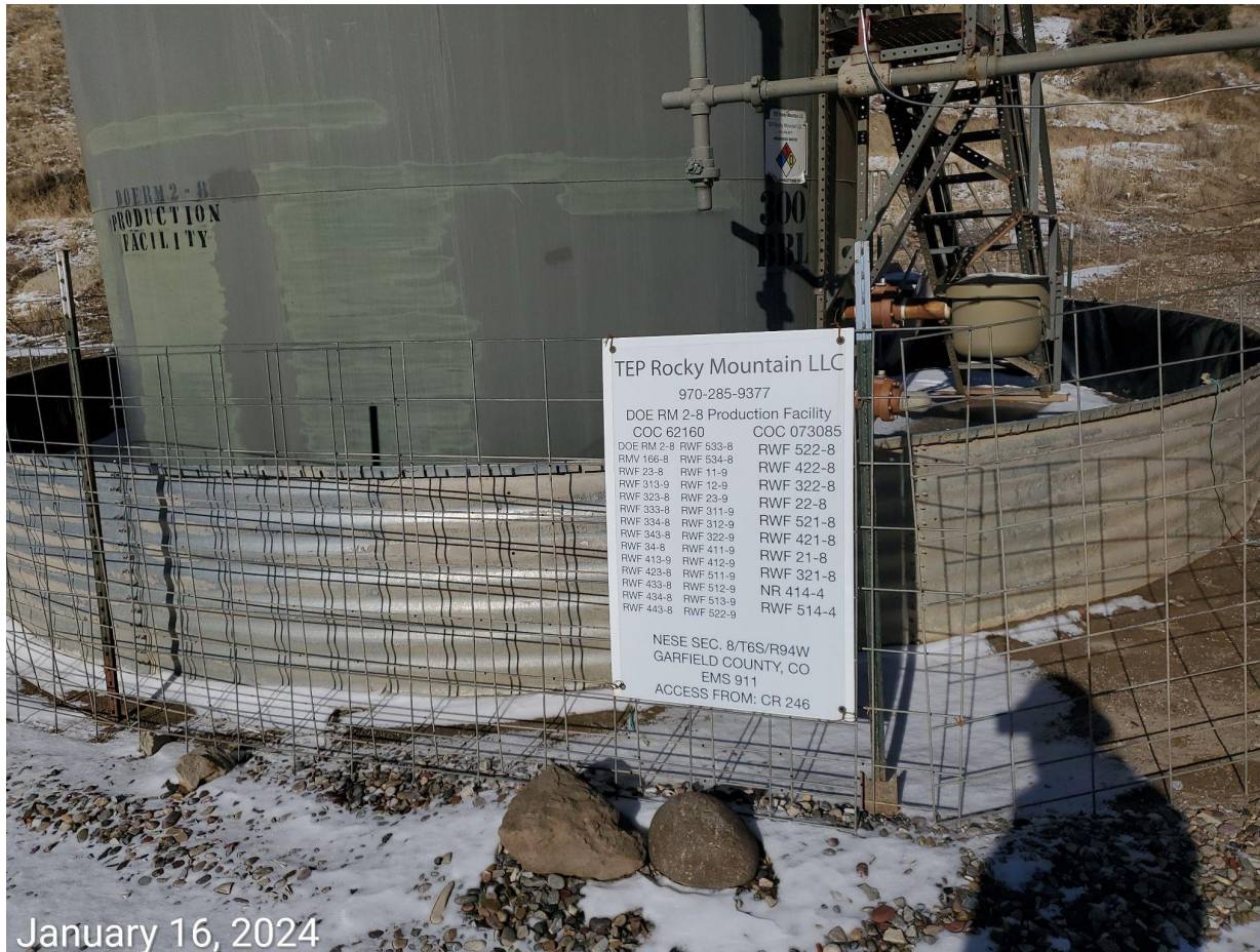
Photo 2: Signage at tank battery missing required well API information.
