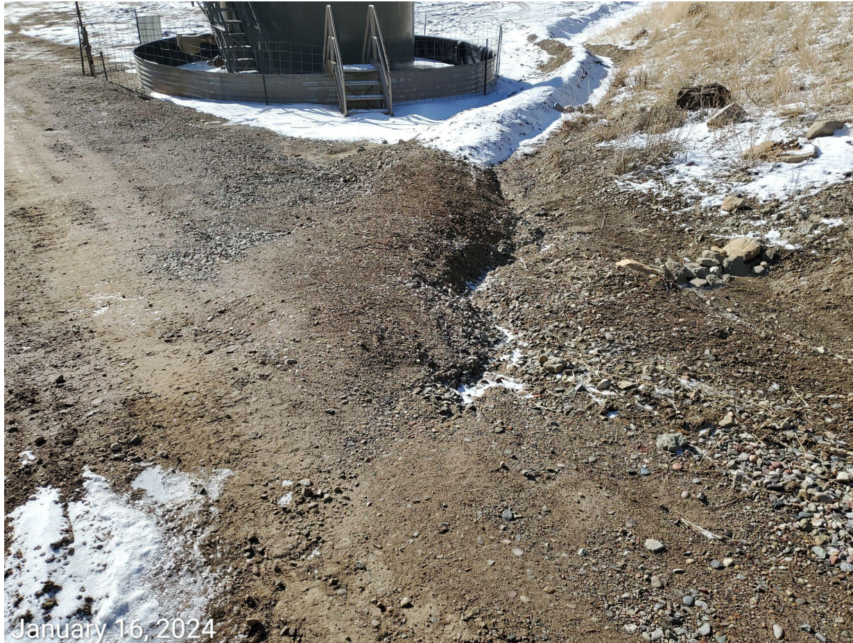
Photo 3: Erosion degradation developing along access road.
