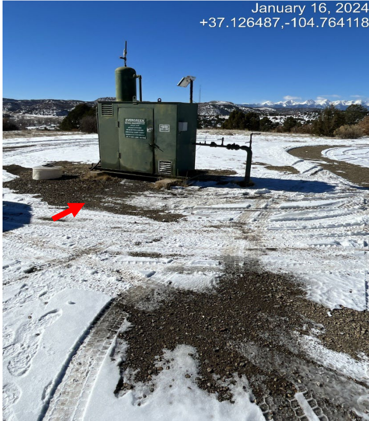
Photo 4. There appeared to have been a leak at meter shed.
