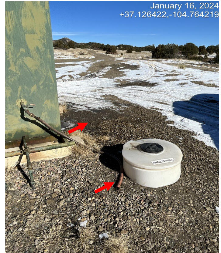
Photo 5. The hose is not placed in the tank.
