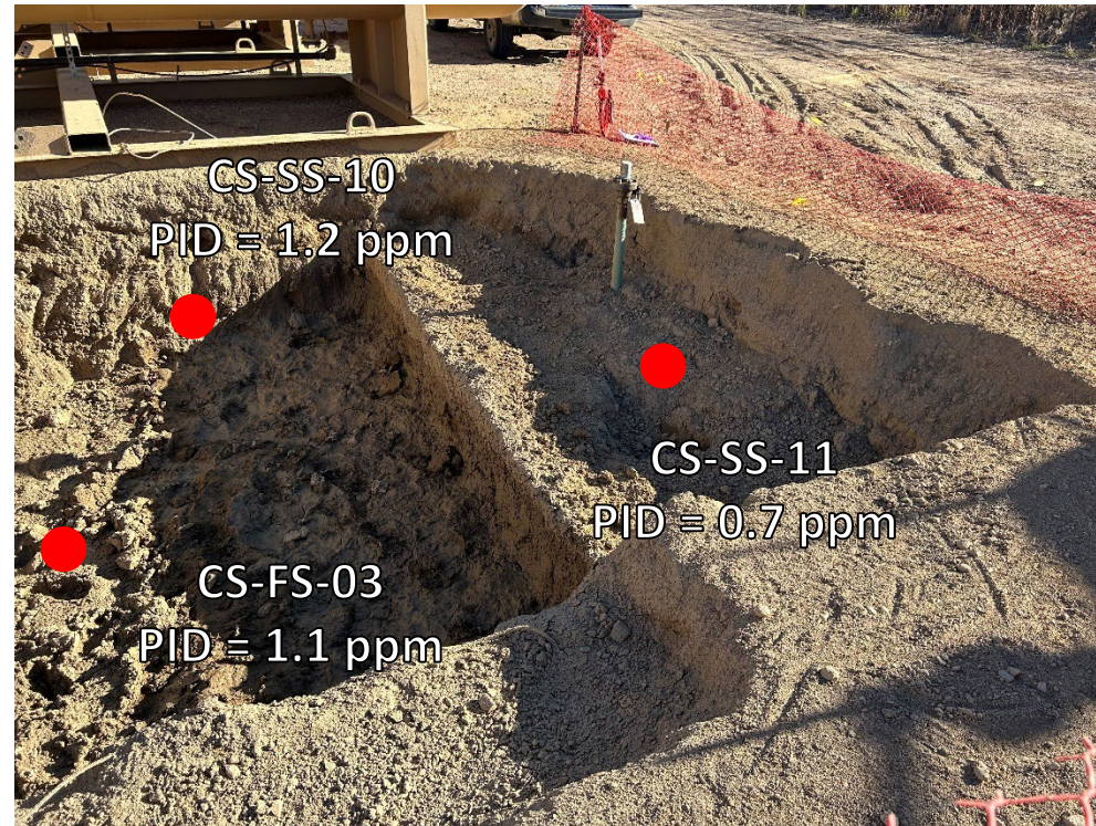
Looking east-northeast at over-excavation of SS-02, SS-13, FS-01, FS-02, CS-SS-04, CS-SS-06
