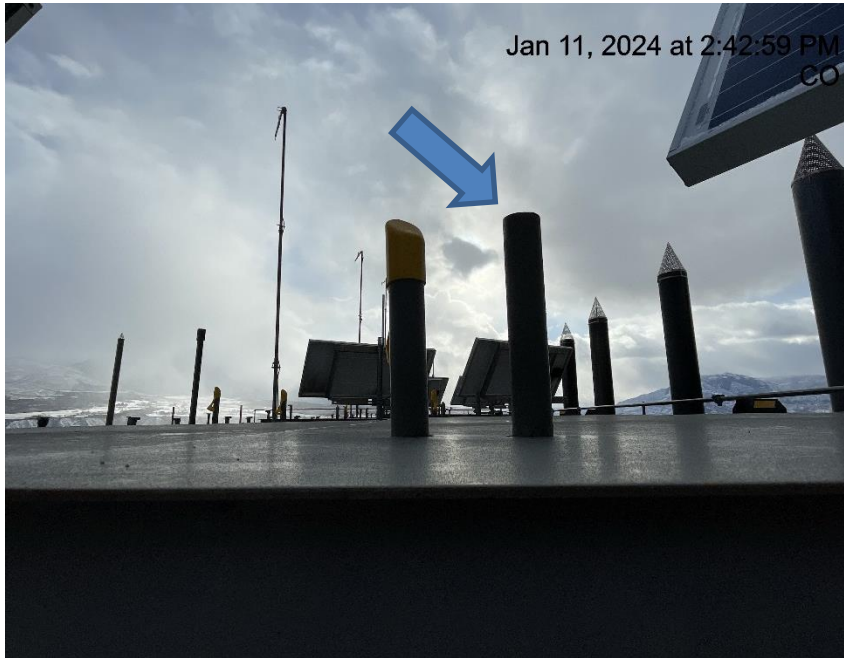
Photo # 2600 PRV vent line lacks cap
