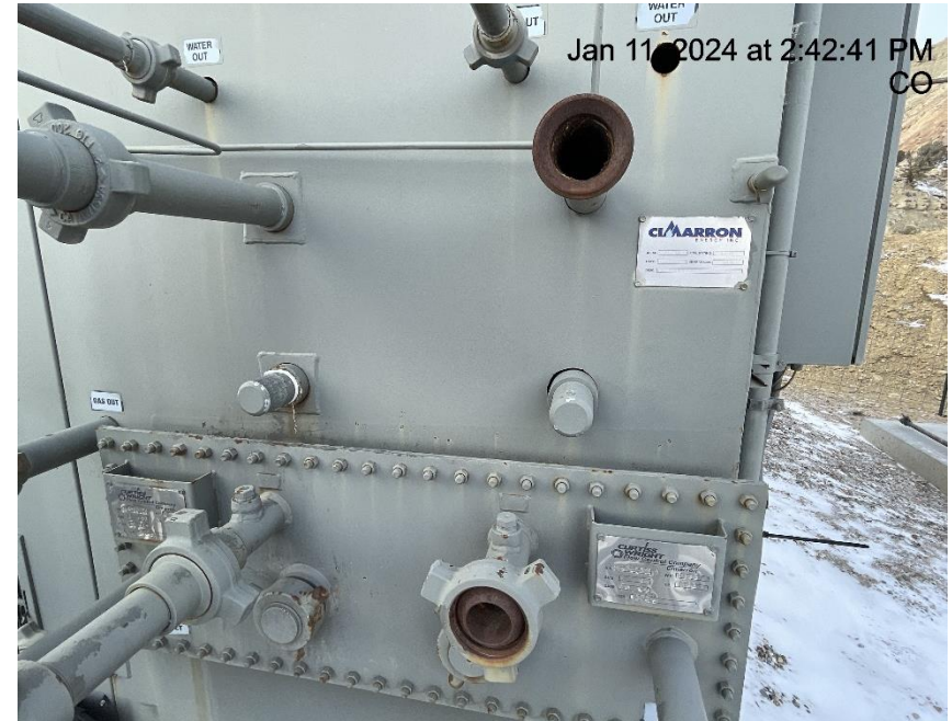
Photo # 2599 Open ended piping/wildlife hazards on separator
