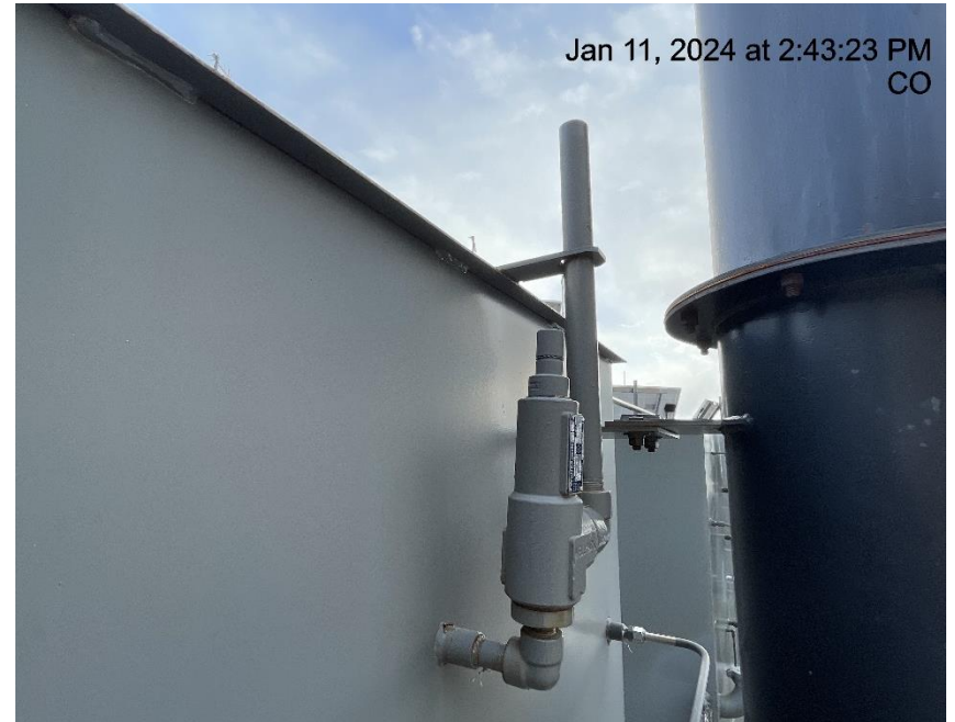
Photo # 2601 PRV vent line lacks cap
